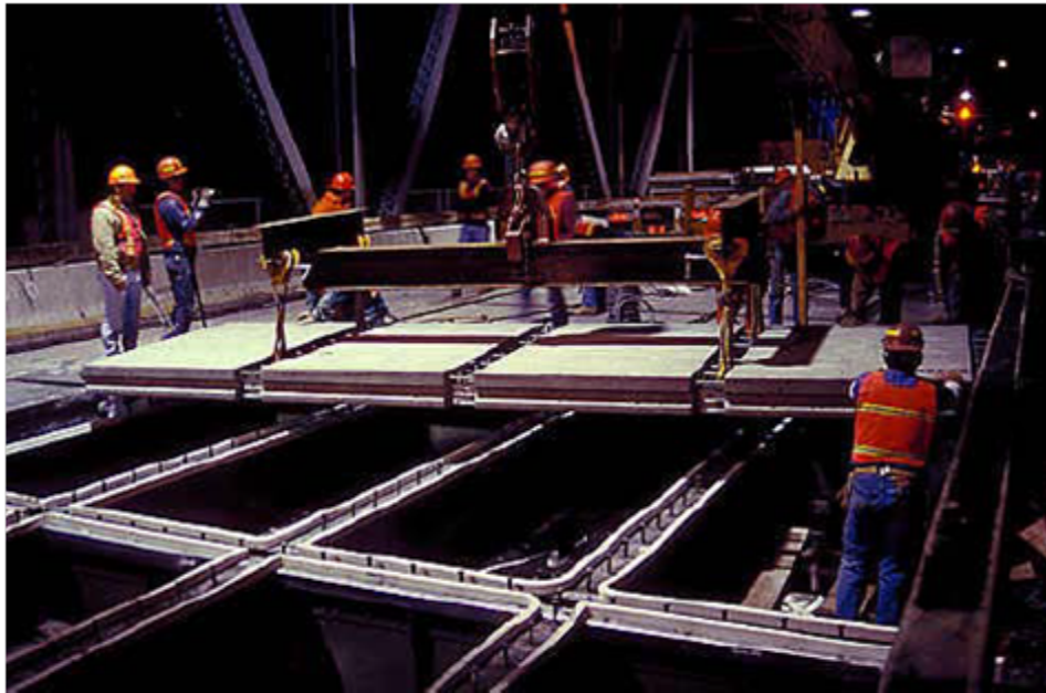
Figure 2.7: Exodermic Deck Installation ( www.fhwa.dot.gov/bridge/prefab/if09010/02.cfm )
