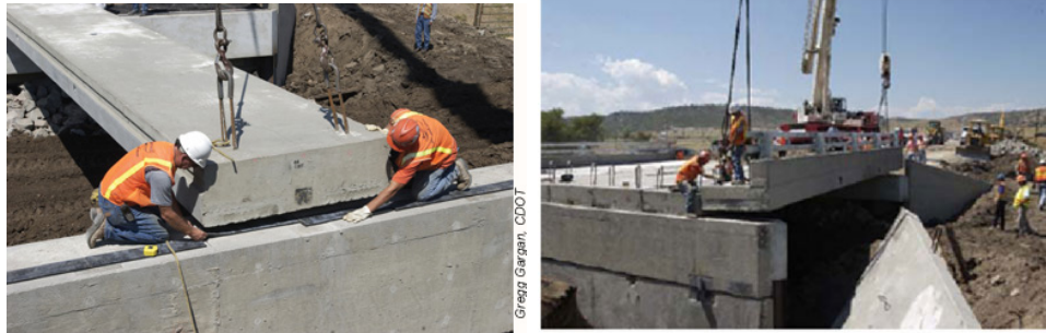
(a) First Beam Being Placed
