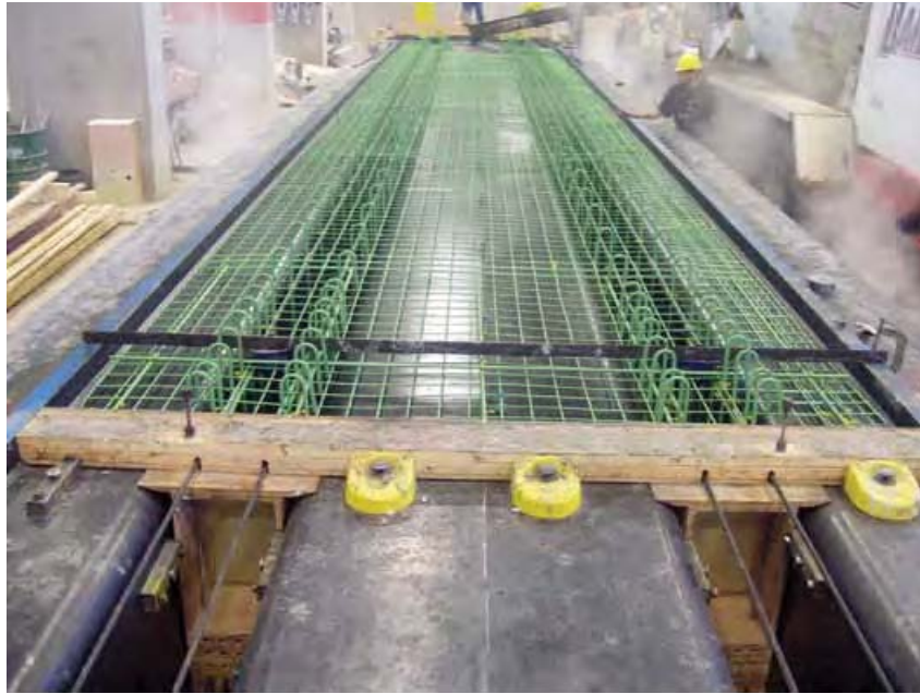
Figure 4.6: NEXT Beam Fabrication ( www.pci.org/view_file.cfm?file=JL-10-SUMMER-9.pdf )
