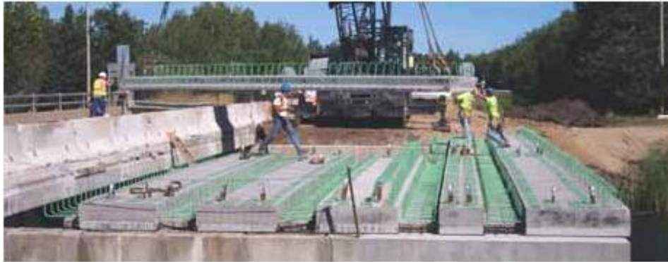
Figure 4.3: Center City Bridge Under Construction ( www.dot.state.mn.us/bridge/manuals/LRFD/pdf/workshop/06InvertedTeeDesign.pdf )
