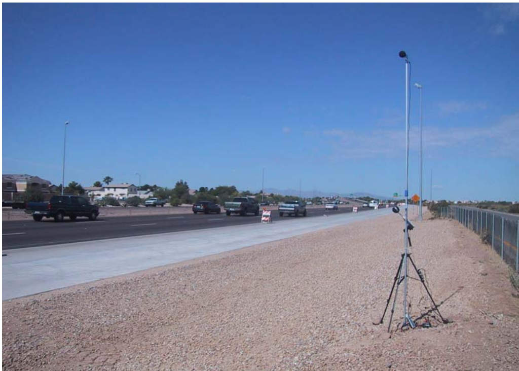
Figure E3: Site 3A Geometry Changes relative to Microphone Locations after Addition of Auxilliary Lane
