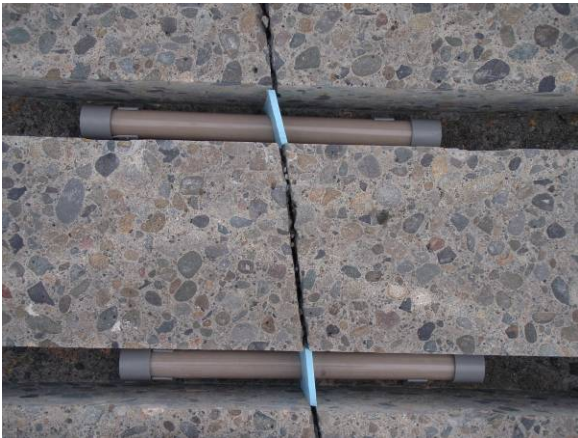
Figure 6. Close-up of dowels in slots.
