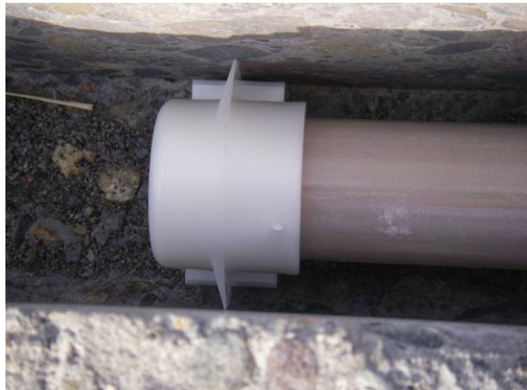
Figure 10. End caps on GFRP dowels.
