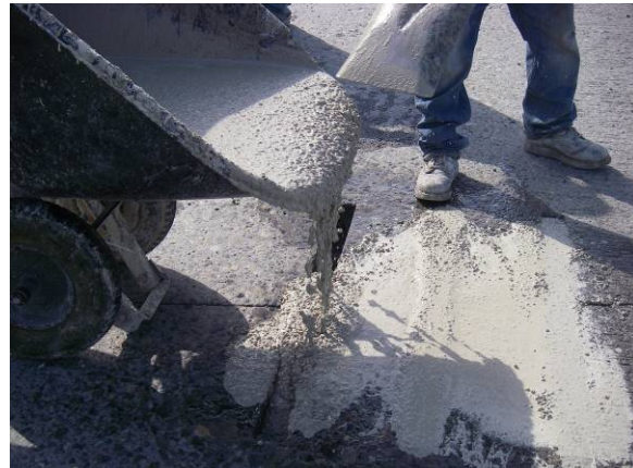
Figure 11. Slot filling.
