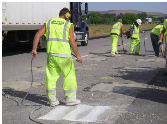
Figure 12. Application of curing compound.
