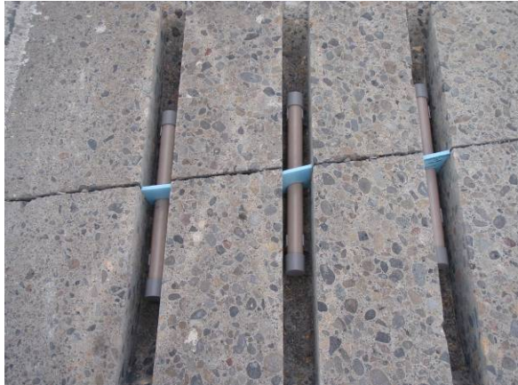
Figure 5. GFRP dowels placed in slots.
