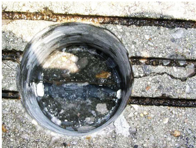
The development of a transverse deck crack, at the right, is examined by taking a core sample.
