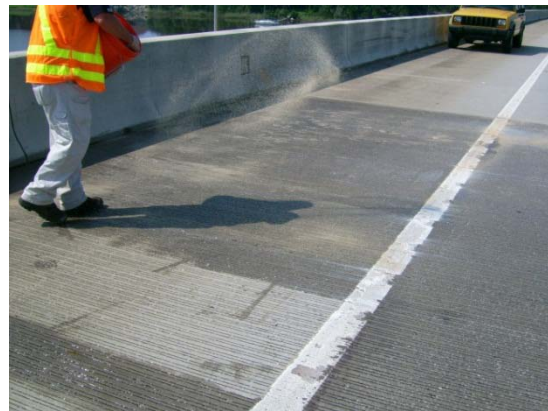
Figure 3-52: Sand spray by hand
