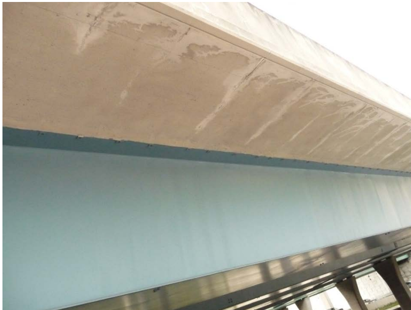
Figure 3-5: Fort Lauderdale Bridge
