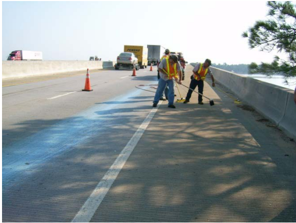
Figure 3-47: Mixing sealer materials
