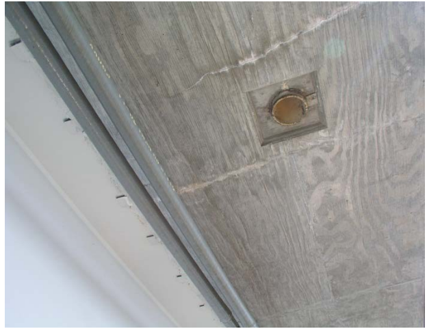
Figure 3-3: Deck and soffit cracking
