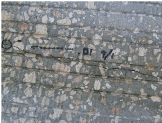
Figure 3-11: Deck cracking and supporting girders
