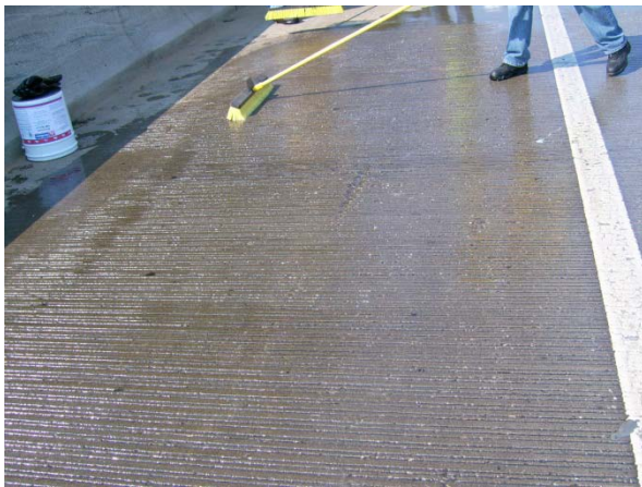
Figure 3-49: Applying sealers to the deck
