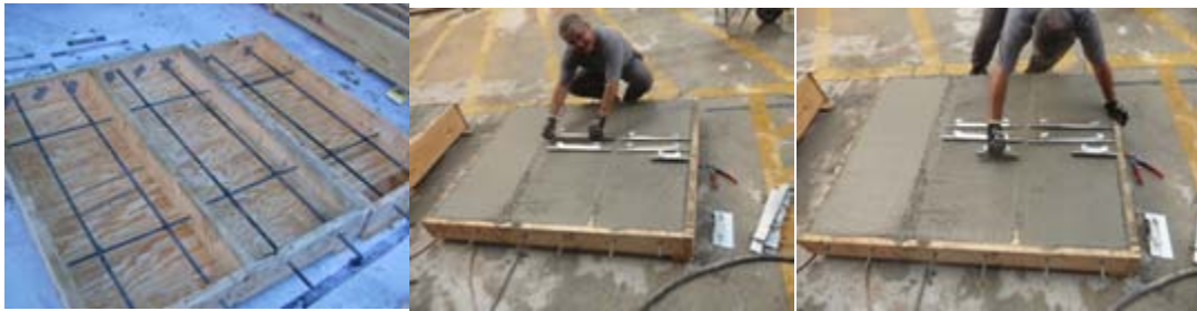
Figure 3-18: Construction of test slabs and placement of blades for crack width
