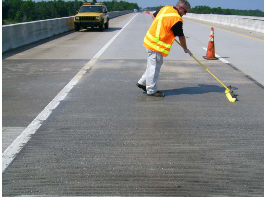
Figure 3-14: Apply sealants to the cracked deck
