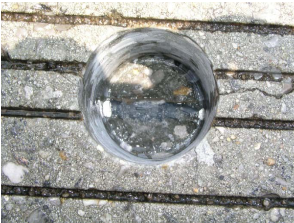
Figure 3-4: Core sampling showing crack development over the transverse reinforcement
