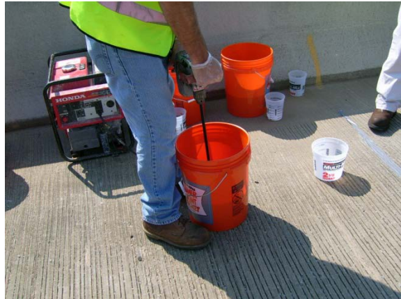
Figure 3-48: Cleaning the cracked deck
