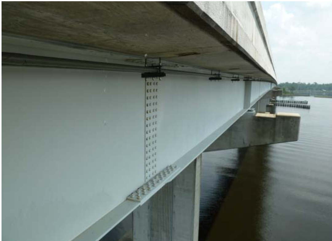
Figure 3-1: Blackwater River Bridge (Milton-Pensacola)
