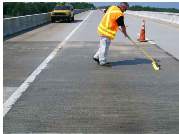
Figure 3-50: Spreading the sealers
