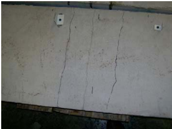
Figure 4-6: Control slab cracking
