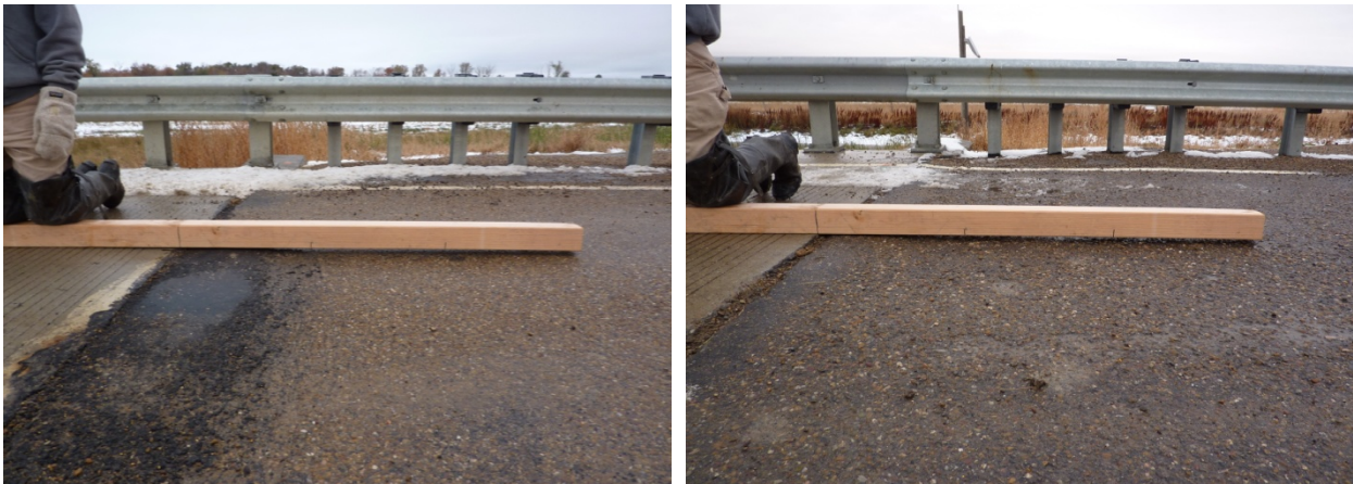
Figure 18: Paved approaches of the HPC deck (NW-left, SE-right) in 2009.
