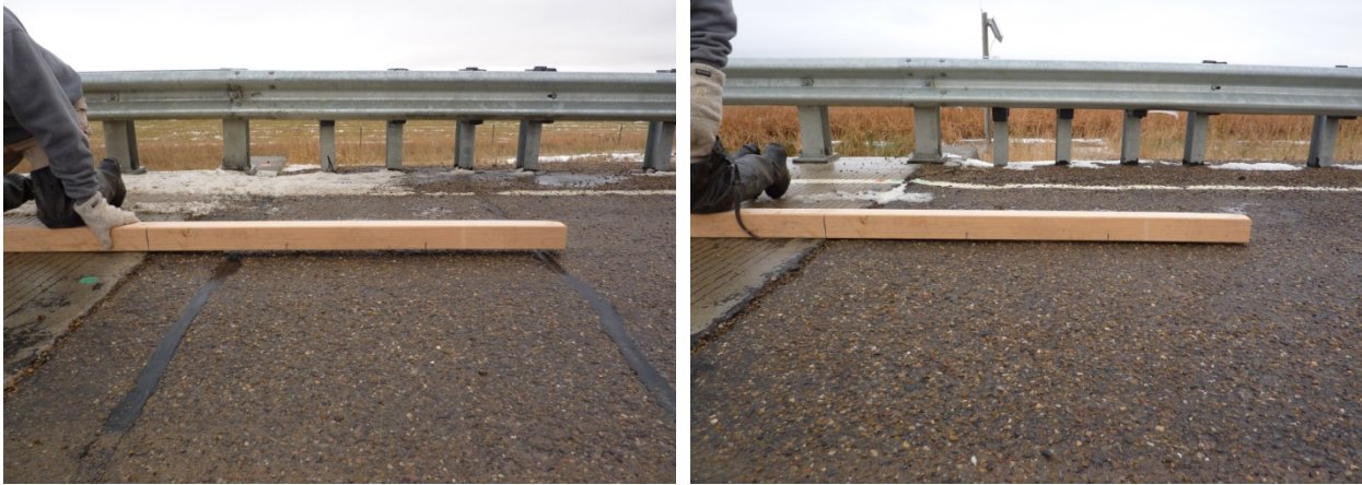
Figure 17: Paved approaches of the Empirical deck (NW-left, SE-right) in 2009.
