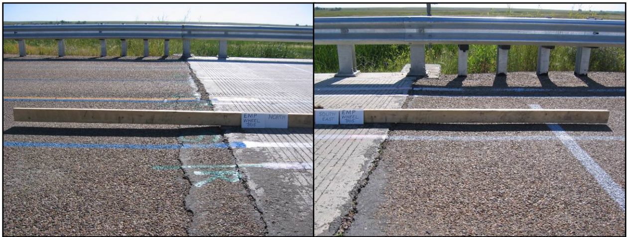
Figure 115: Paved Approaches of the Empirical Deck (NW-left, SE-right)
