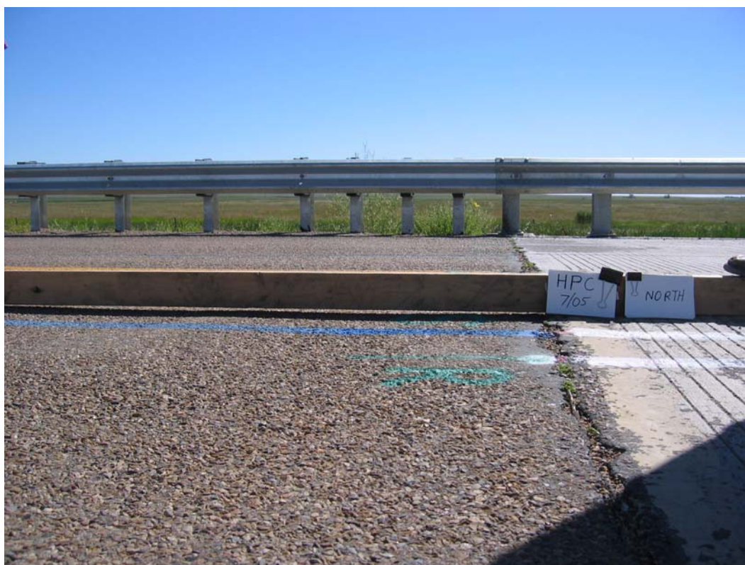
Figure H -32: Paved Approach – Northwest End of HPC Deck
