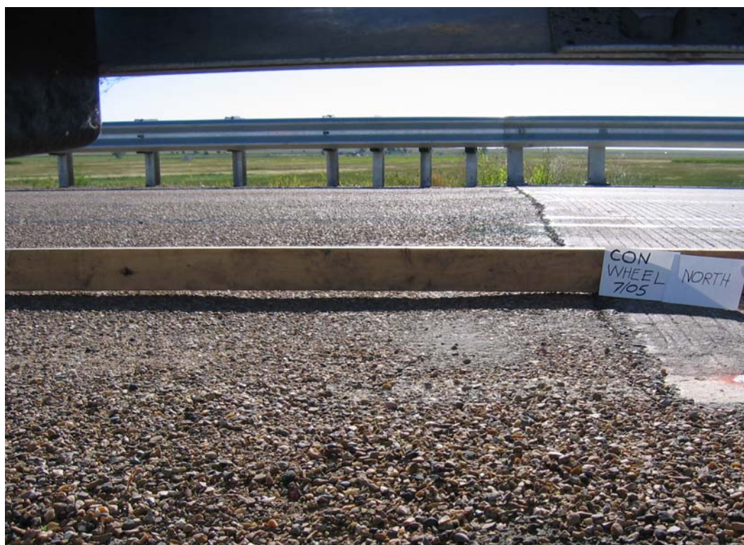
Figure H -8: Paved Approach – Northwest End of Conventional Deck
