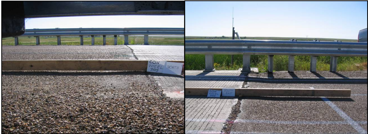
Figure 114: Paved Approaches of the Conventional Deck (NW-left, SE-right)
