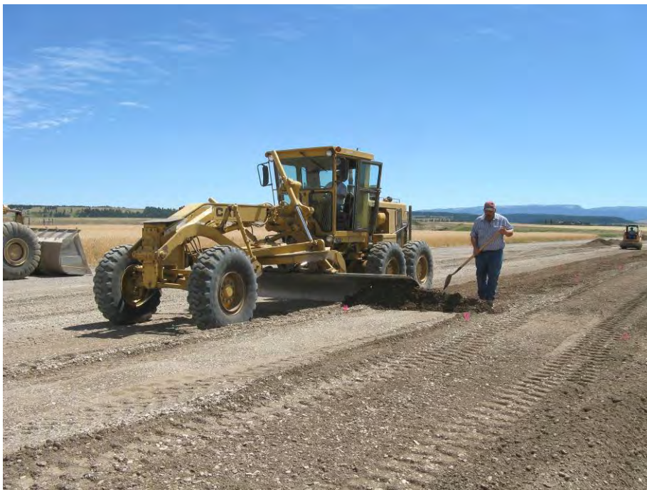
Figure 28. Final grading of the base course surface.
