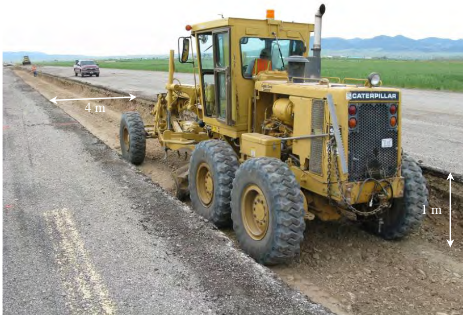
Figure 13. Final grading of the test pit.
