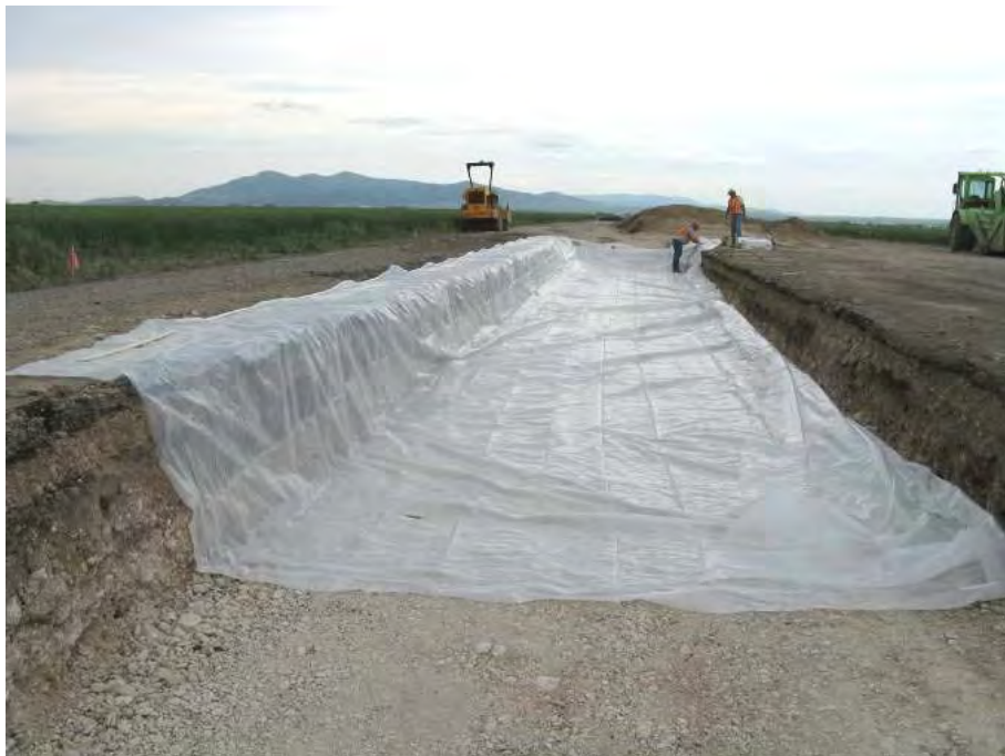
Figure 14. Installation of plastic liner in test pit.
