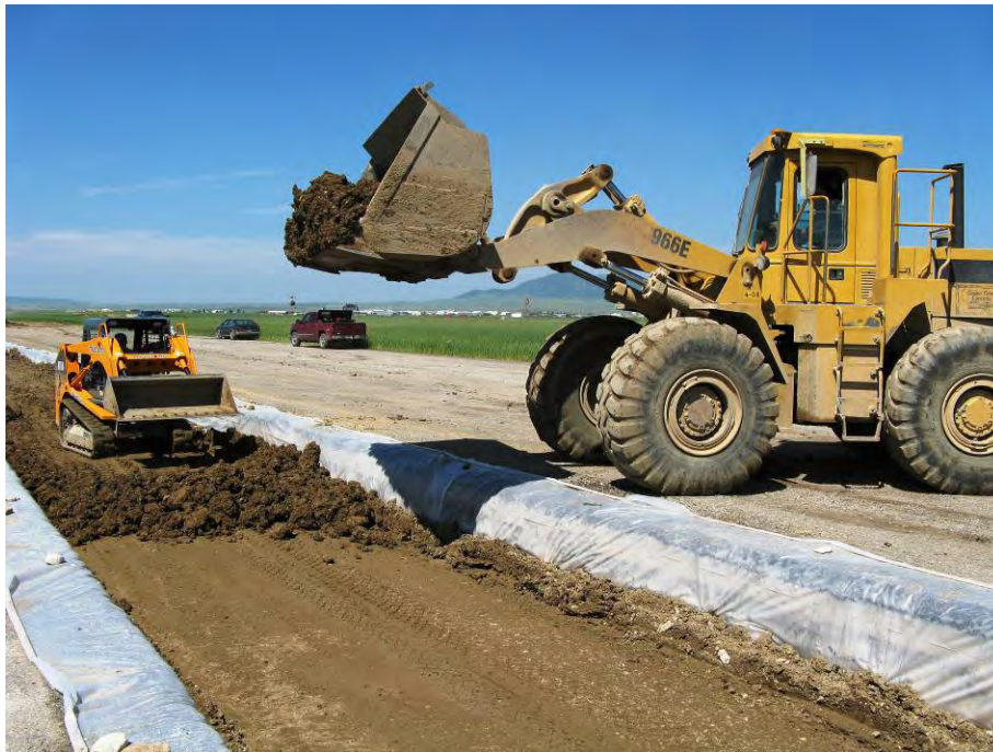
Figure 15. Delivery and distribution of the artificial subgrade in the test pit.
