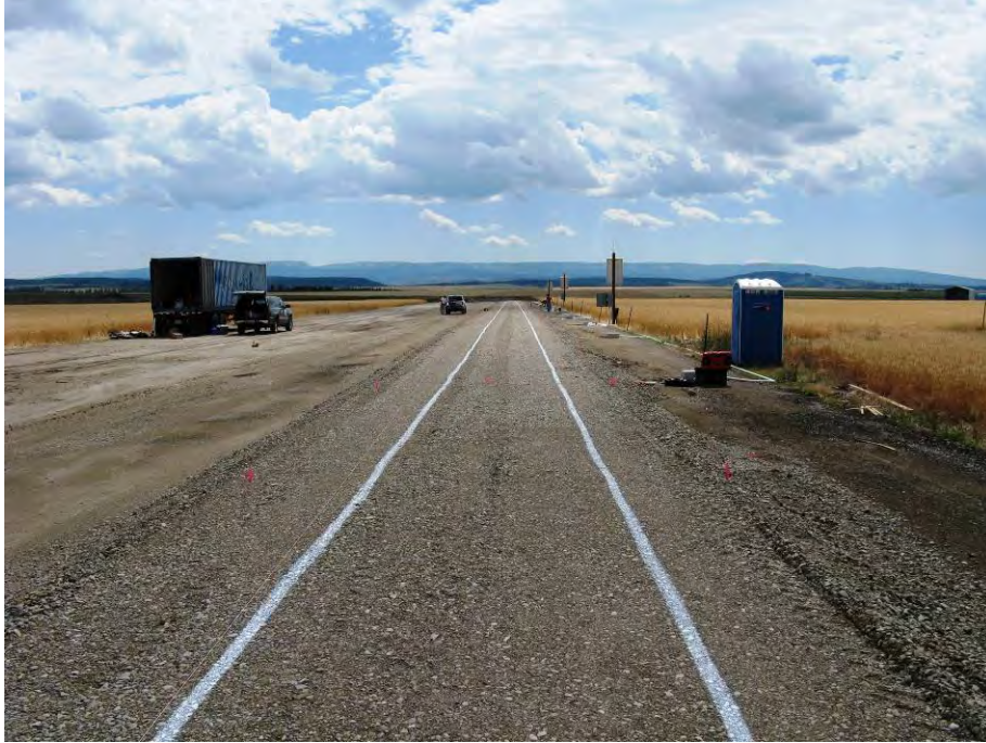
Figure 33. Full view of test area prior to trafficking.
