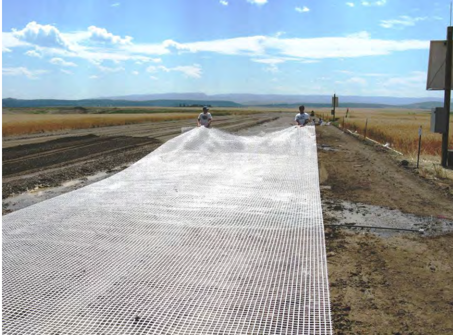
Figure 26. Installation of geosynthetics.
