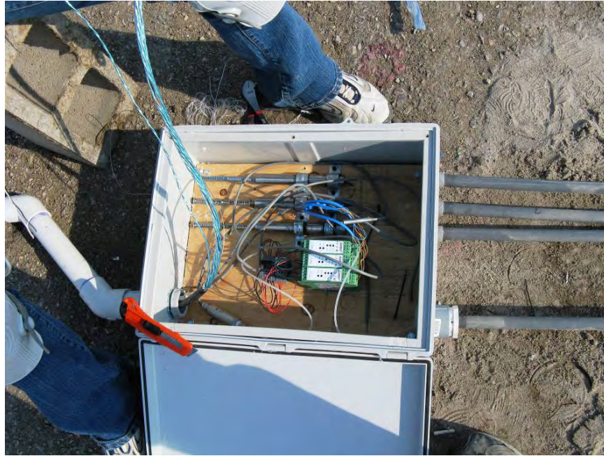
Figure 8. Installation of sensor box.
