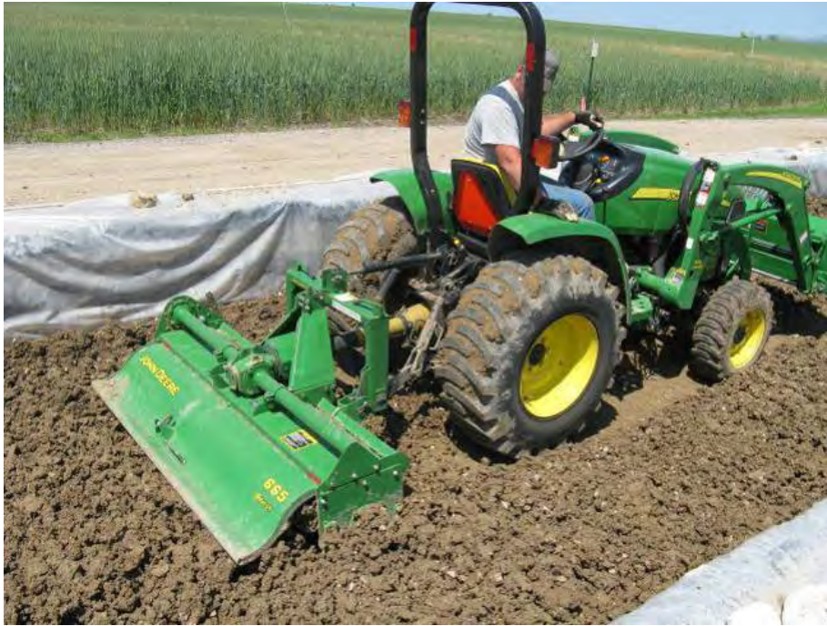
Figure 16. Mixing the subgrade layer with large roto-tiller.
