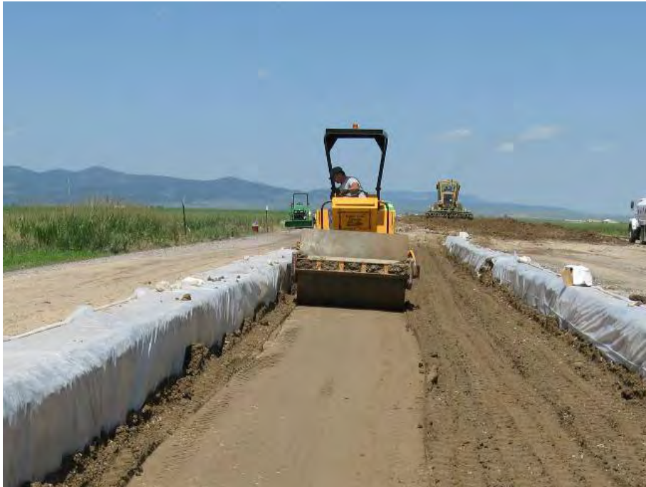
Figure 17. Compacting subgrade with smooth drum, vibratory roller.
