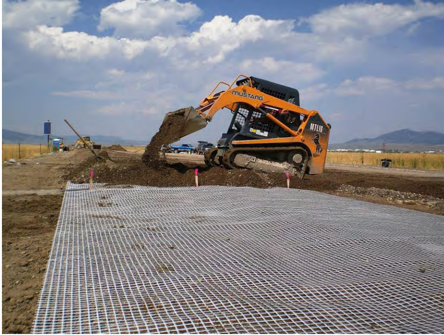
Figure 27. Placement of base course aggregate.
