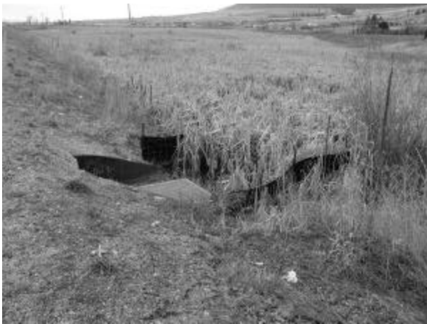
West entrance heavily vegetated
