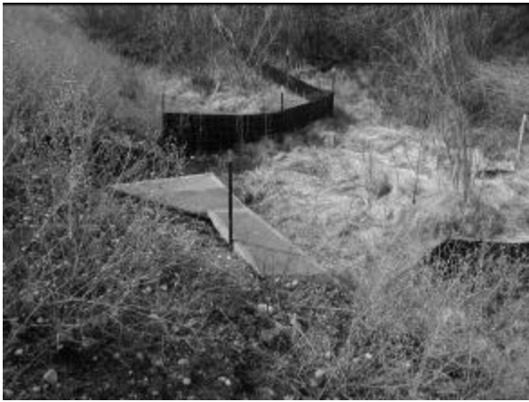
West entrance heavily vegetated
