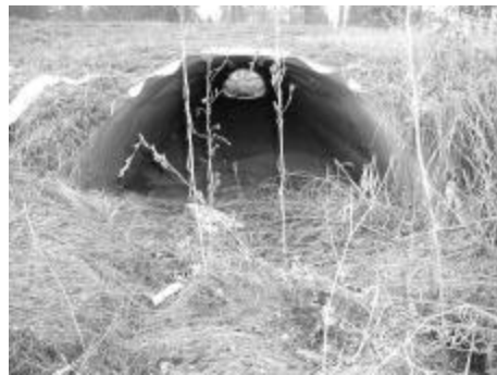
Figure 34. Additional culvert added along Highway 203: Florence culvert.
