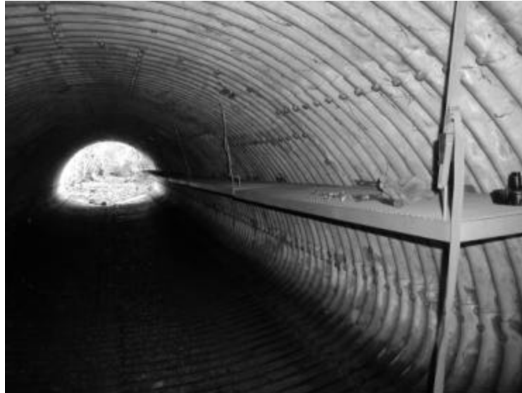
Figure 22. Modified animal shelf placed in Bass Creek Large culvert.
