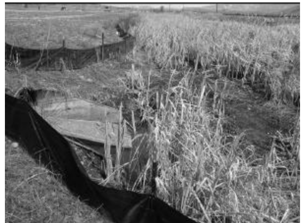
East entrance heavily vegetated
