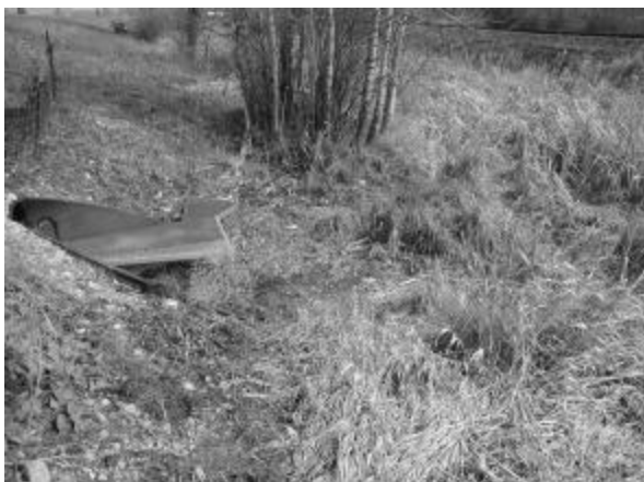
West entrance heavily vegetated
