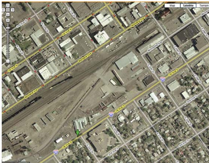
Figure 51: Satellite View of the Billings Intermodal Terminal with Several Cars Lined Up for Loading (Google Maps).
