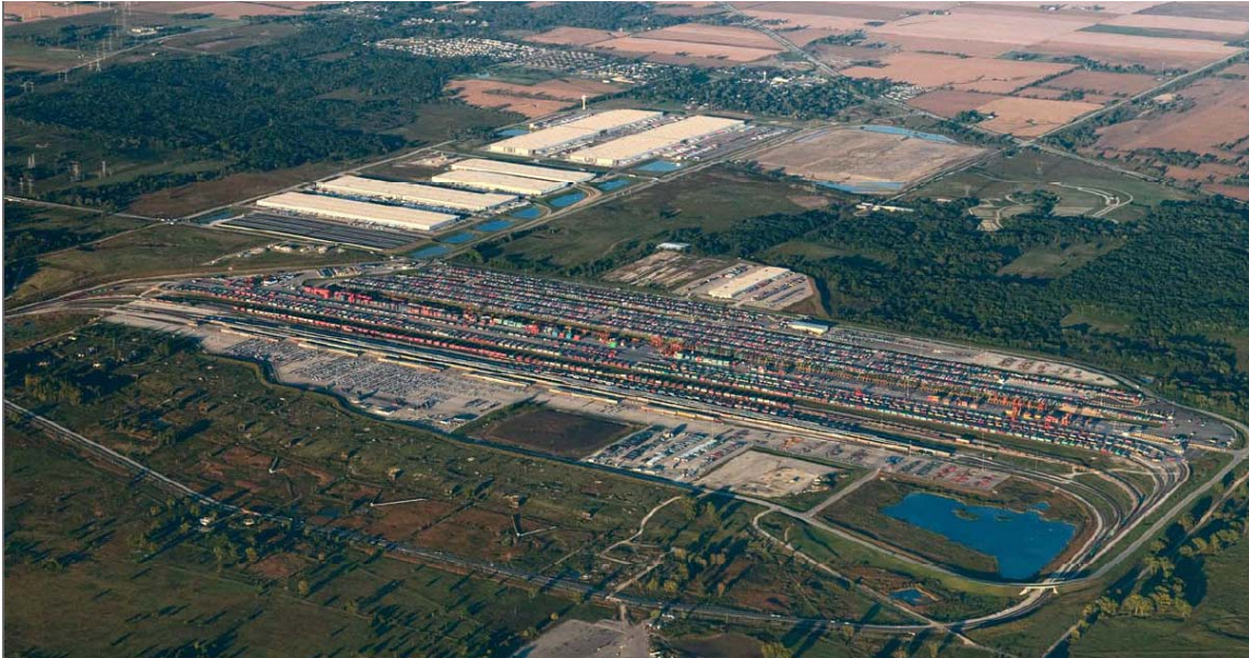
Figure 25: Joliet Intermodal Complex (KACOT 2007).
