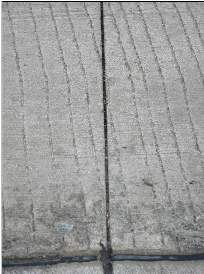
Figure 13. Clean shallow saw cut (Test Cell 3, joint 15 @ 1.00 inch).
