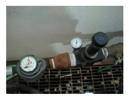
Figure 5. Pressure regulator and flow meter to measure inflow into the rainfall simulator.
