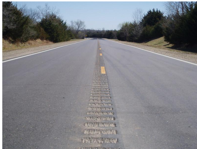
FIGURE 2.7 Centerline Rumble Strips in Kansas
