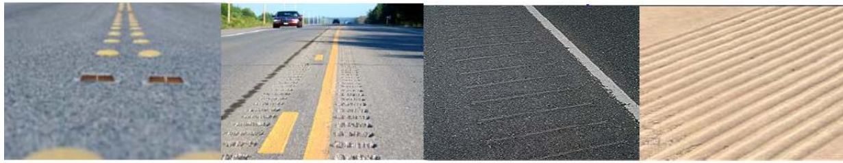
a) Raised b) Milled c) Rolled d) Formed (Source: Richards and Saito, 2005)
