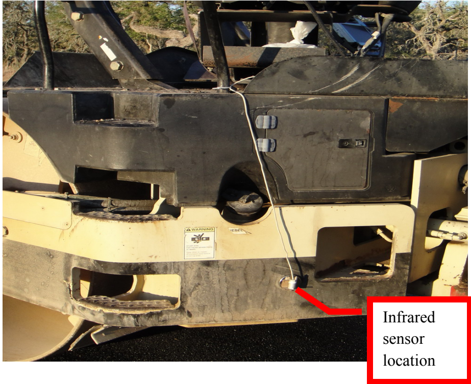
Figure 5. Infrared Sensor Installation.
