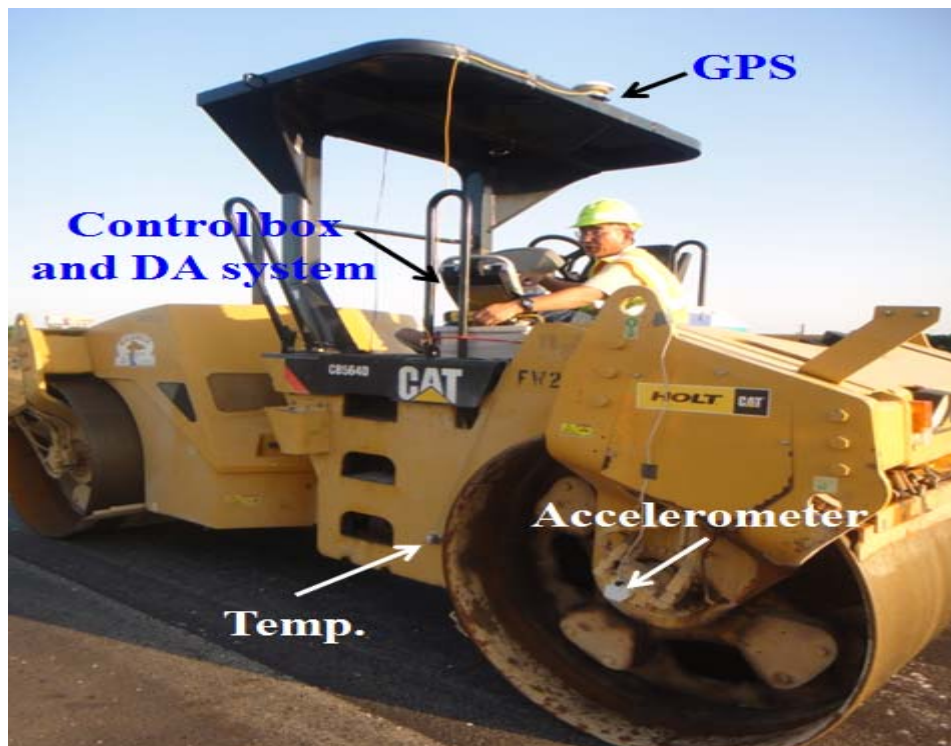
Figure 3. TTI's Complete Compaction Monitoring System.
