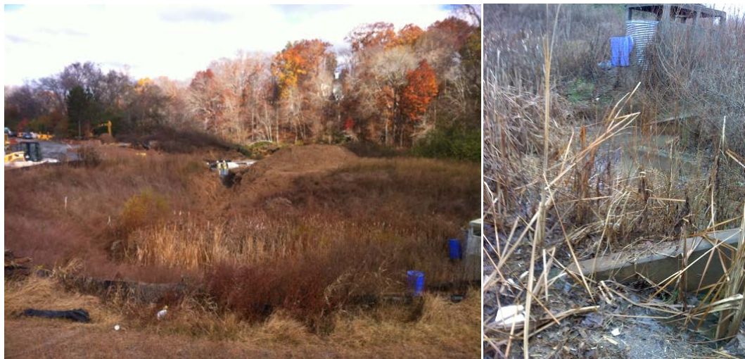
Figure 86. Construction activity and decaying vegetation at McGinnis Ferry BMP.
