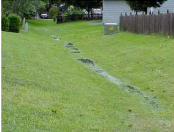
Figure 11. Grass swale. (Georgia Stormwater Manual).
