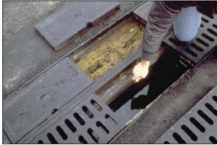
Figure 7. Perimeter sand filter (Georgia Stormwater Manual).
