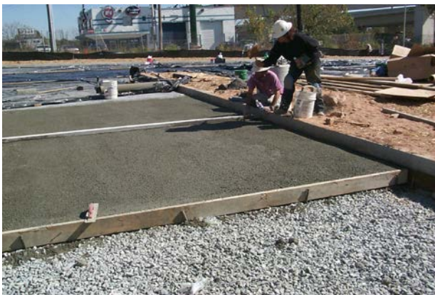
Figure 12. Porous concrete installation (Georgia Stormwater Manual).
