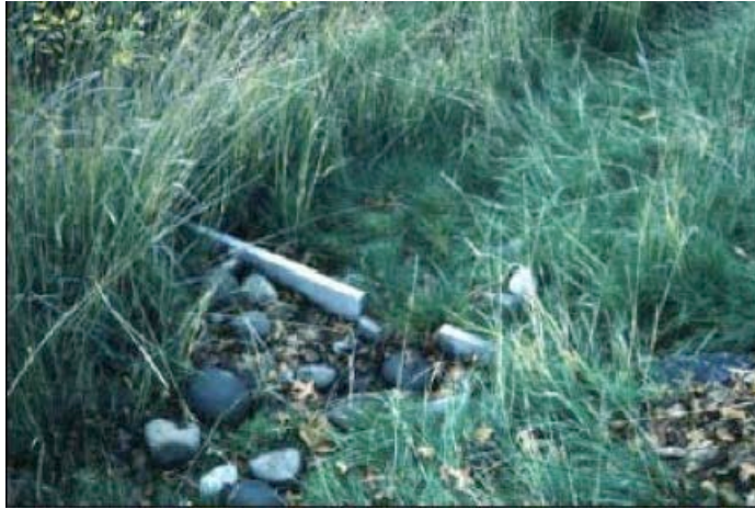
Figure 10. Dry swale (Georgia Stormwater Manual).
