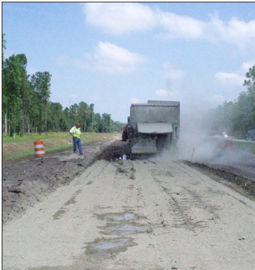
Figure 3-28: Spreading the cement in Test Section 4
