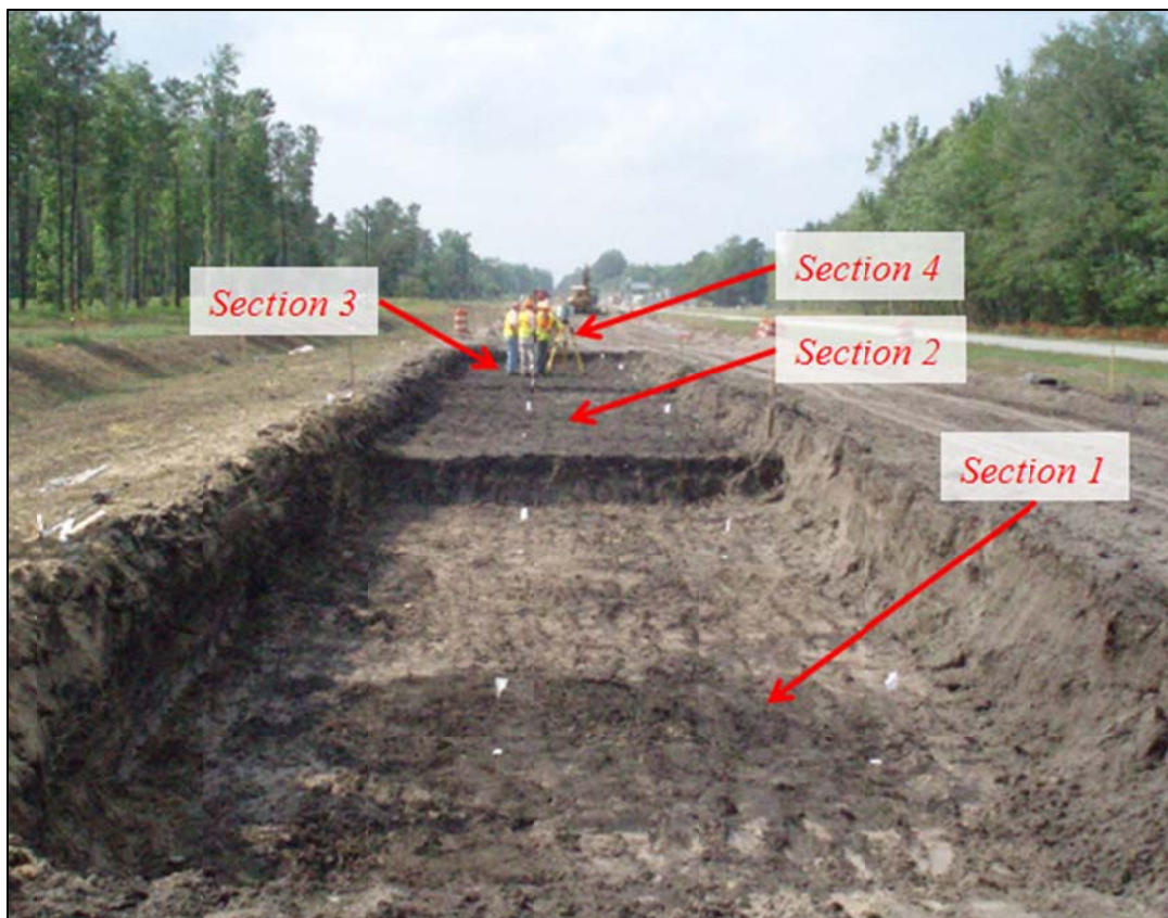
Figure 3-21: Test Sections 1, 2, and 3 undercut to their respective depths
