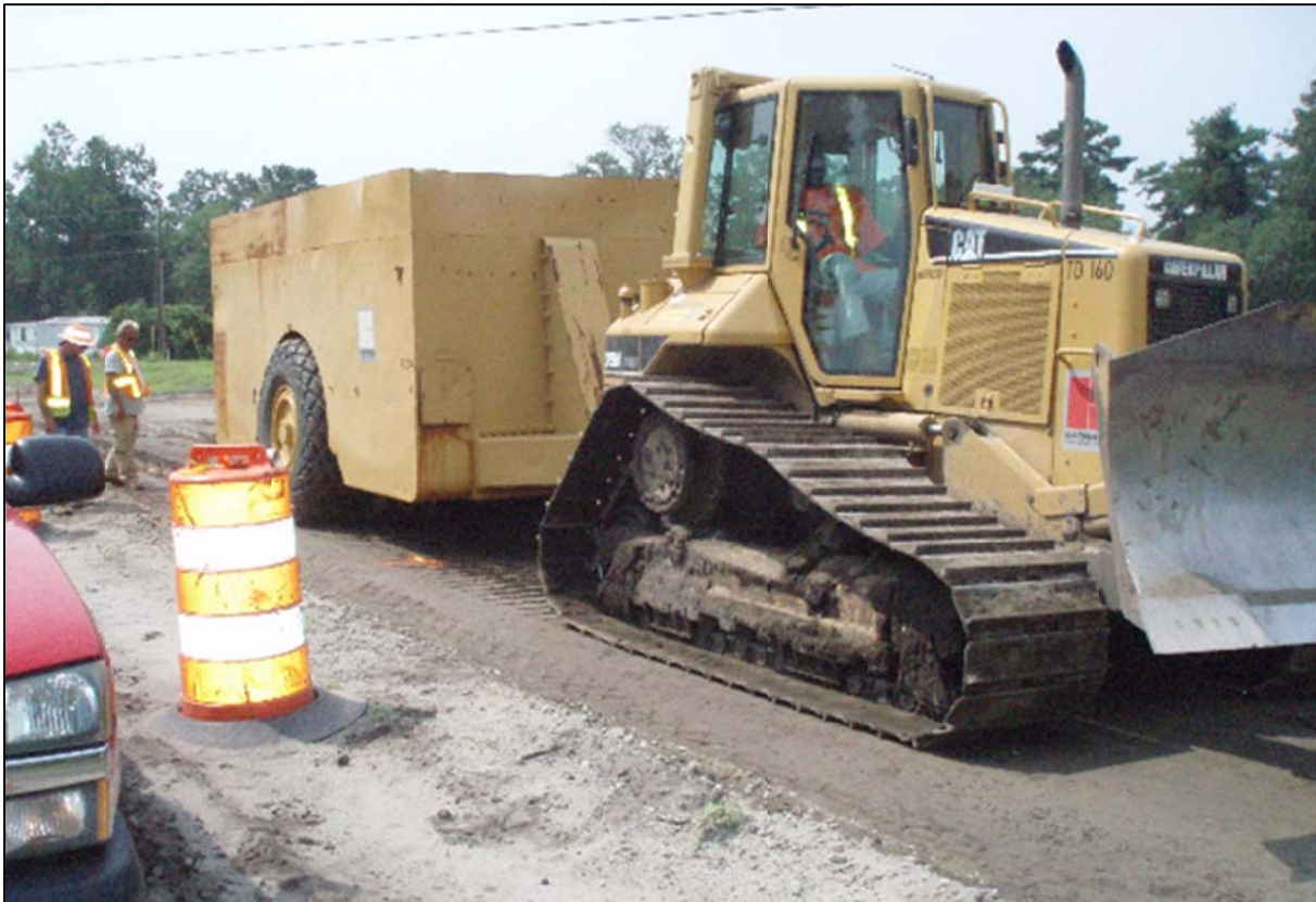
Figure 3-36: Proof rolling performed with 35 ton proof roller
