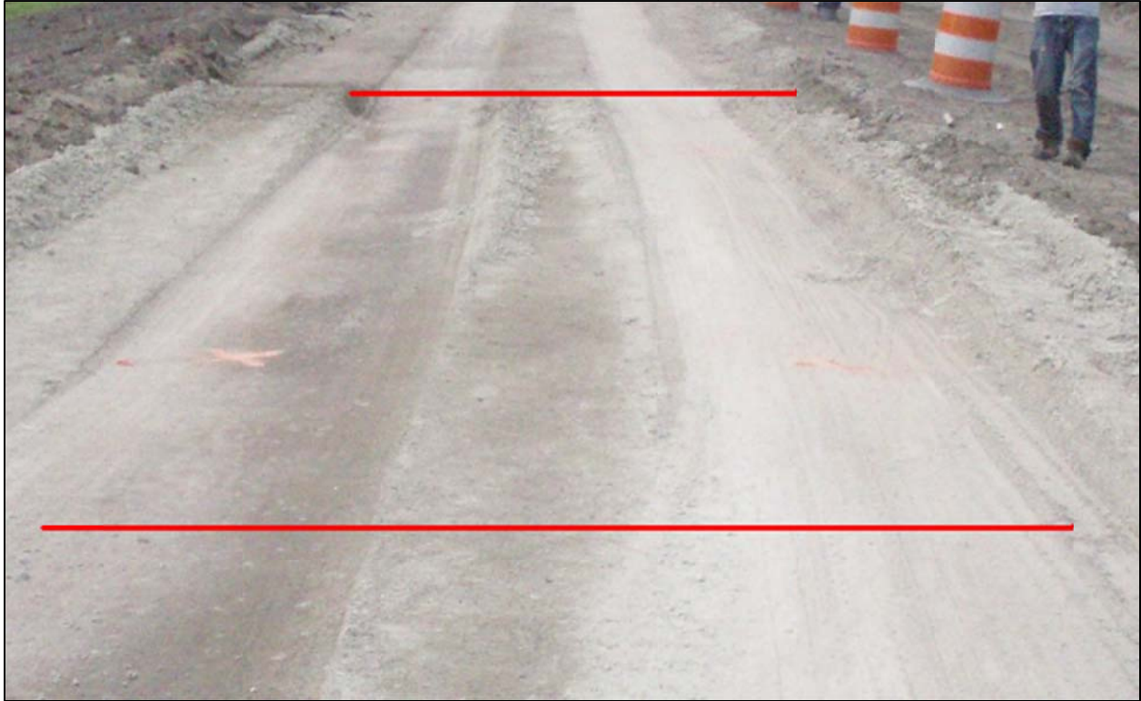
Figure 5-77: Test Section 1 after 1000 truck passes
