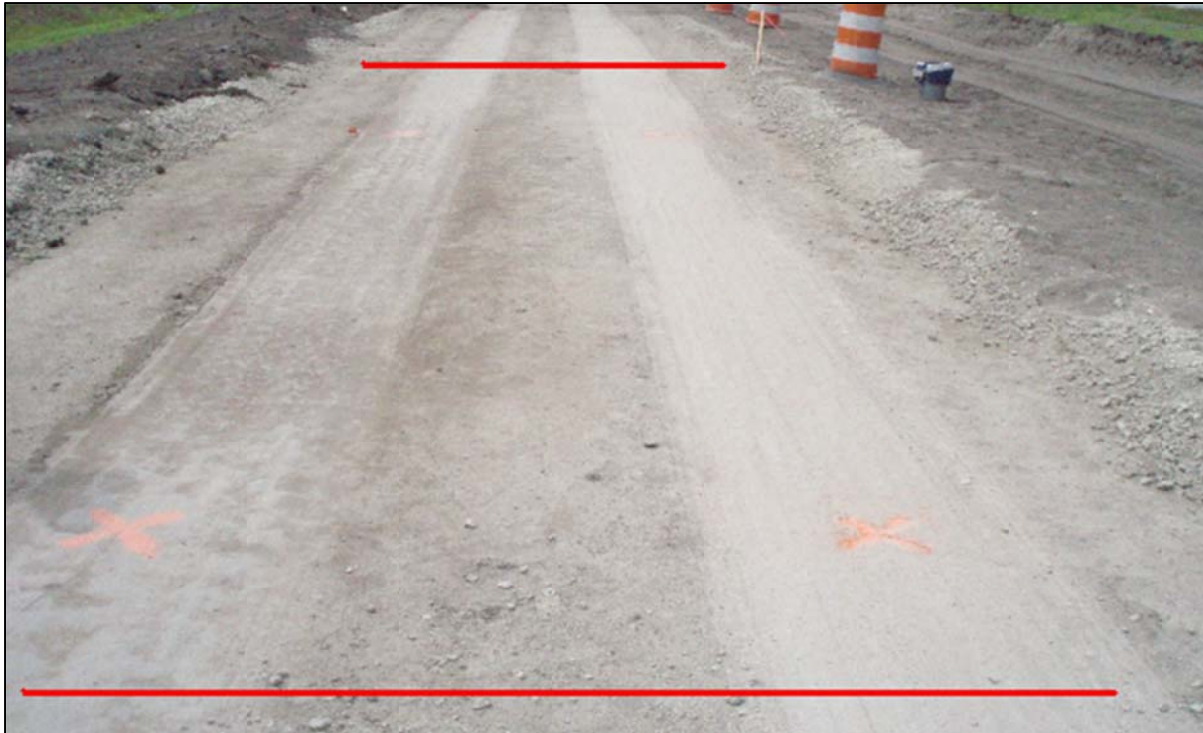
Figure 5-78: Test Section 2 after 1000 truck passes
