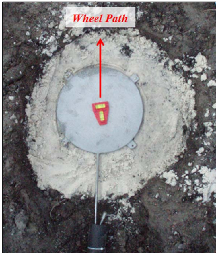
Figure 3-23: EPC installation in Test Section 1
