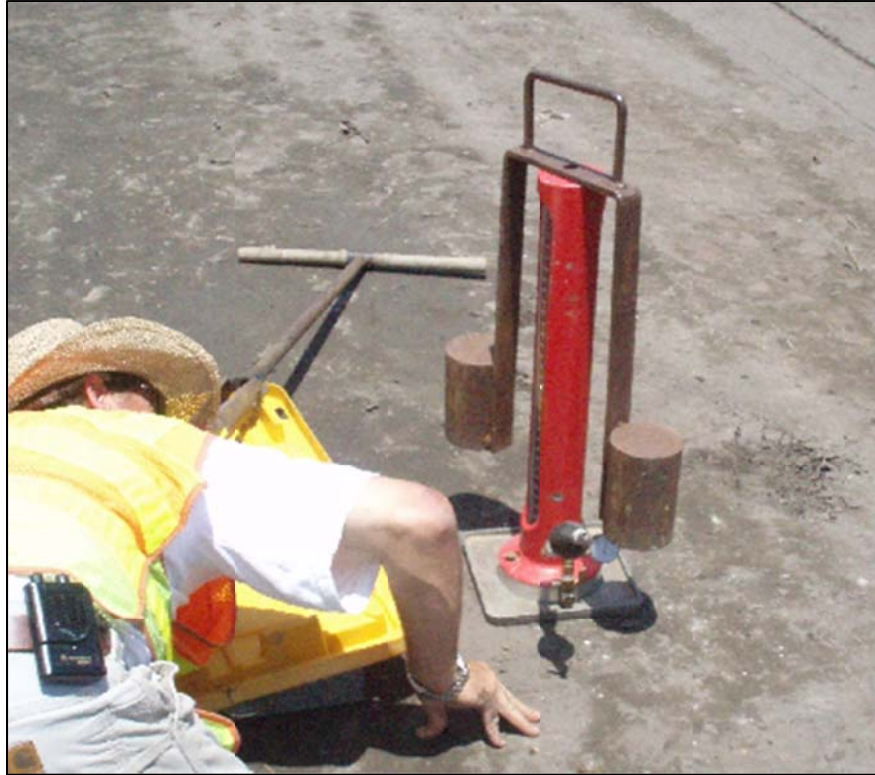
Figure 3-30: Rubber Balloon testing in Test Section 4
