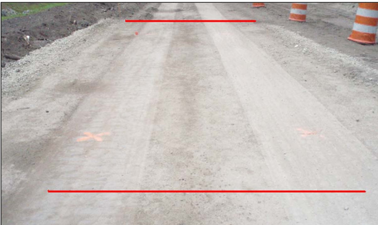
Figure 5-79: Test Section 3 after 1000 truck passes
