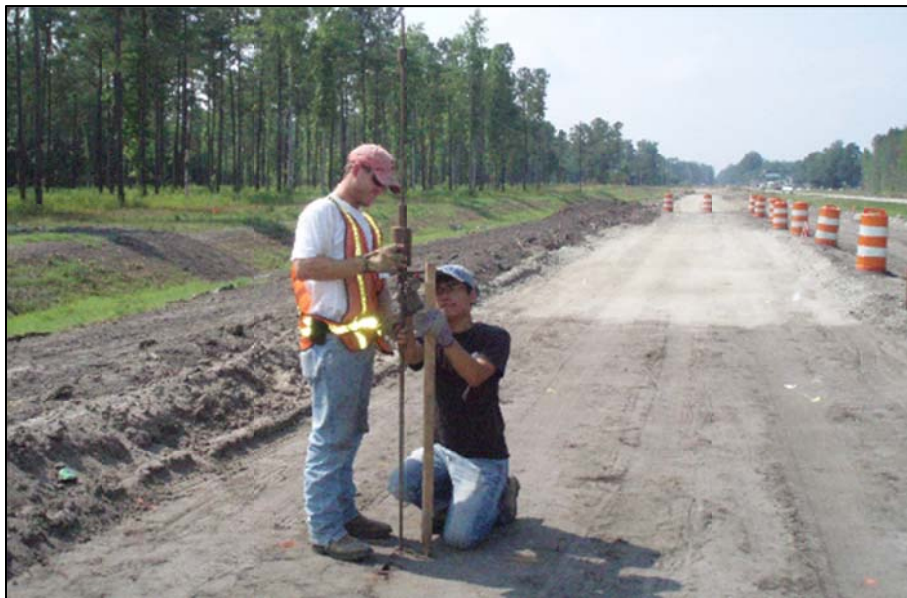
Figure 3-31: DCP testing prior to full-scale testing
