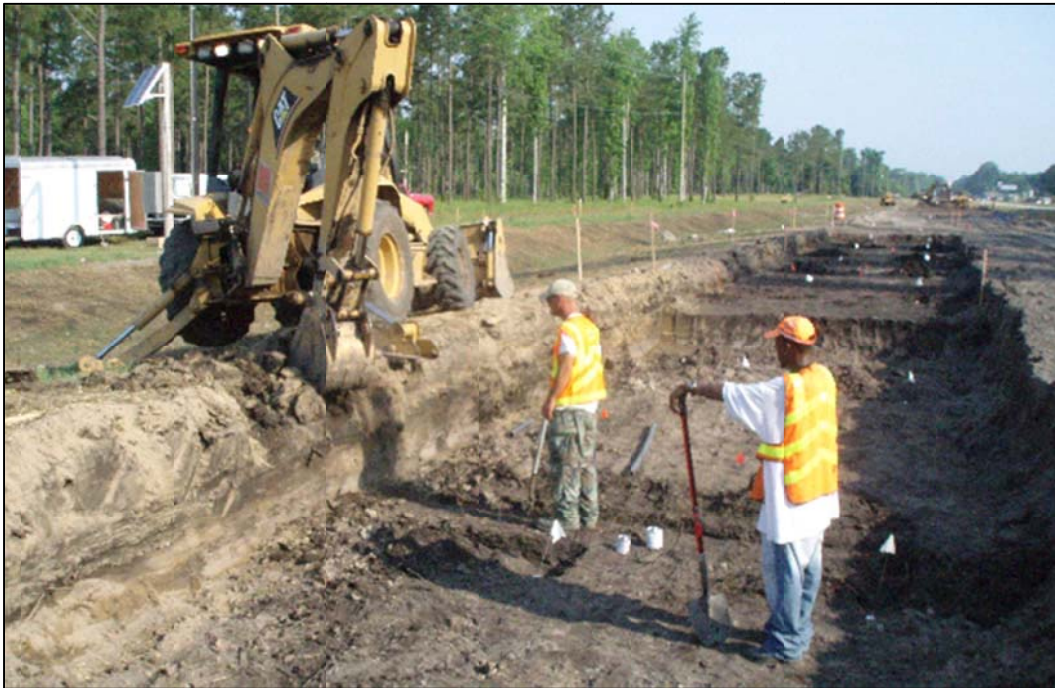
Figure 3-22: Digging trenches for sensor installation in Test Section 1
