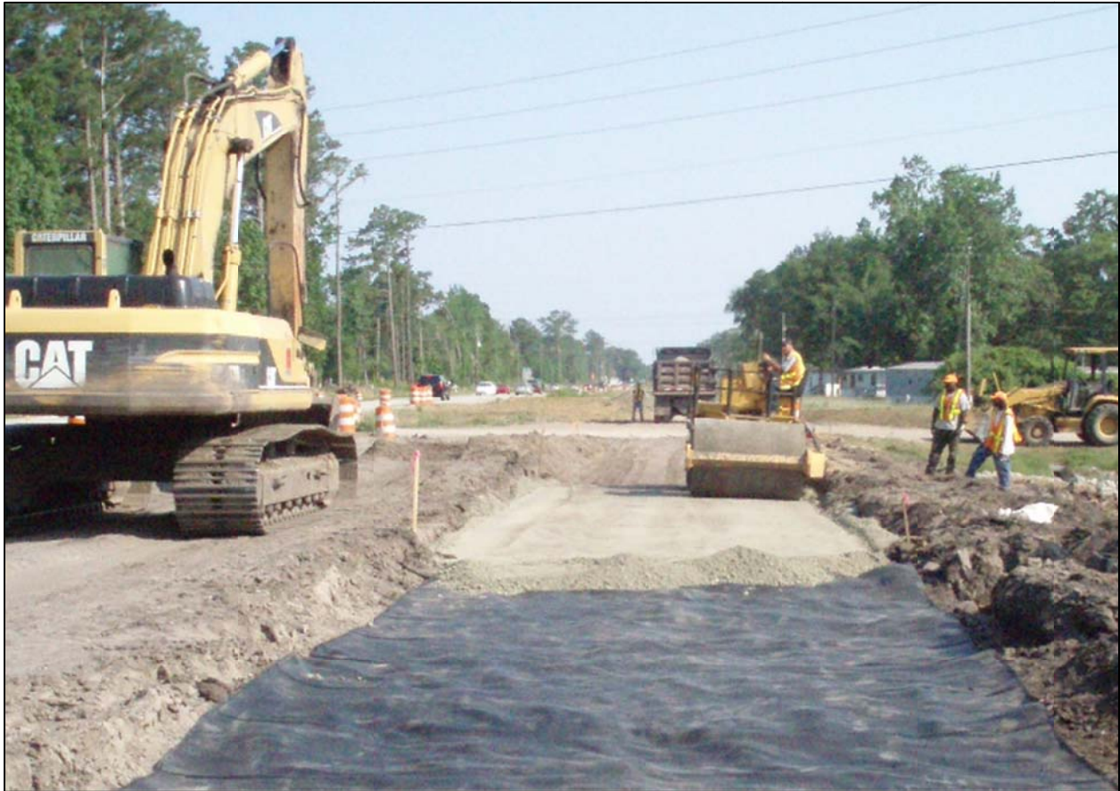
Figure 3-27: Compacting Test Sections 1 and 2 using a steel drum vibratory roller
