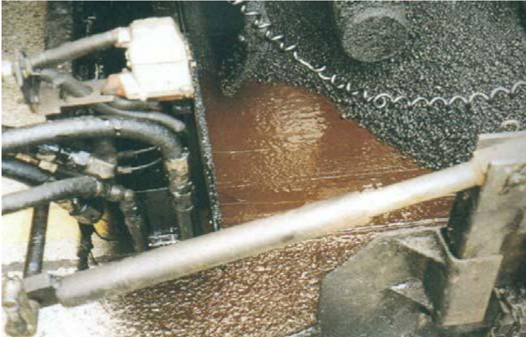
Figure 2.2 Emulsion Membrane and HMA Mix Spreading (Caltrans, 2003)
