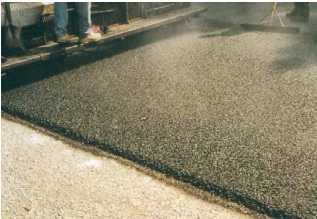
Figure 2.3 Freshly Laid NovaChip (Caltrans, 2003)
