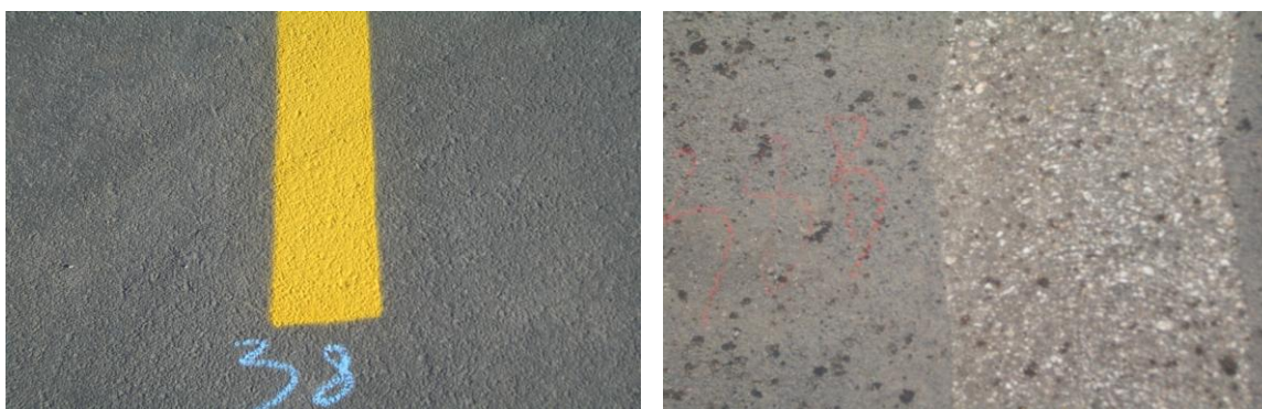
Figure 6.15 Concrete pavement condition before (left) and after (right) 12 mils paint has been removed by PCD grinder
