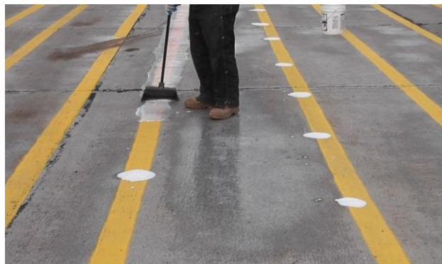
Figure 6.16 Applying the chemicals on the markings
