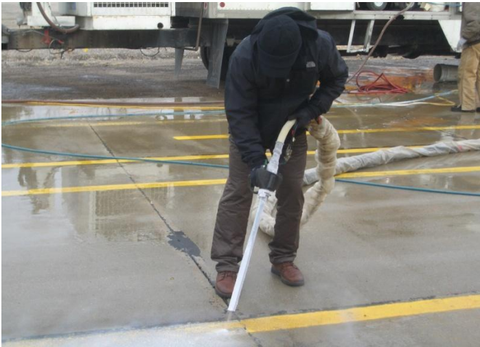
Figure 6.6 Dry ice is shot onto the markings
