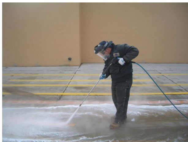
Figure 6.17 Operator with proper protection while removing marking by chemical method
