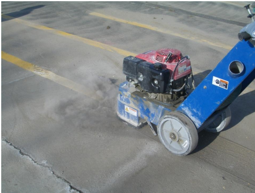
Figure 2.3 Grinder removing paint on asphalt pavement
