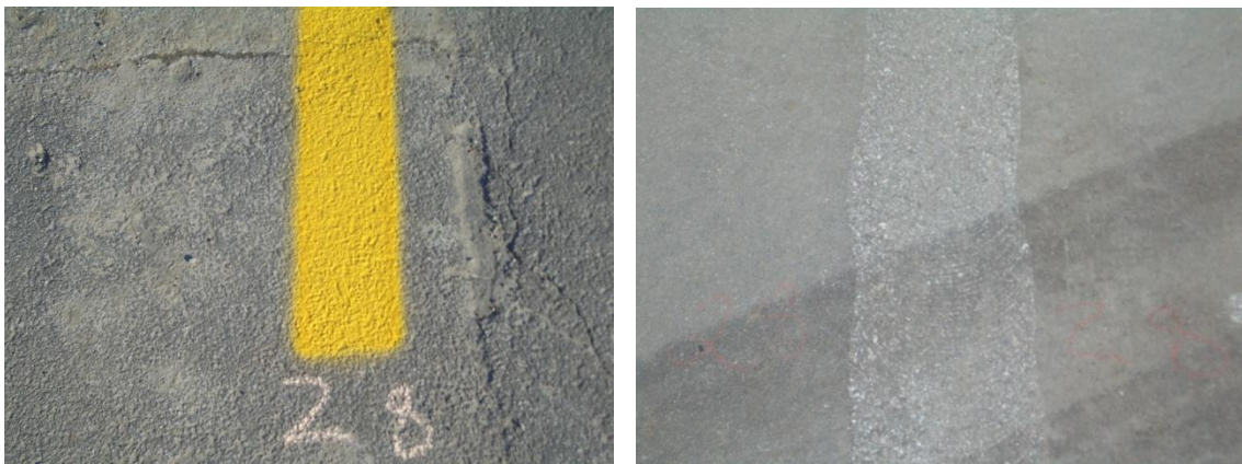
Figure 6.11 Asphalt pavement condition before (left) and after (right) paint has been removed by grinding
