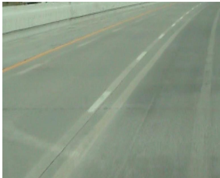
Figure 2.1 Scars on I-80 that can confuse drivers
