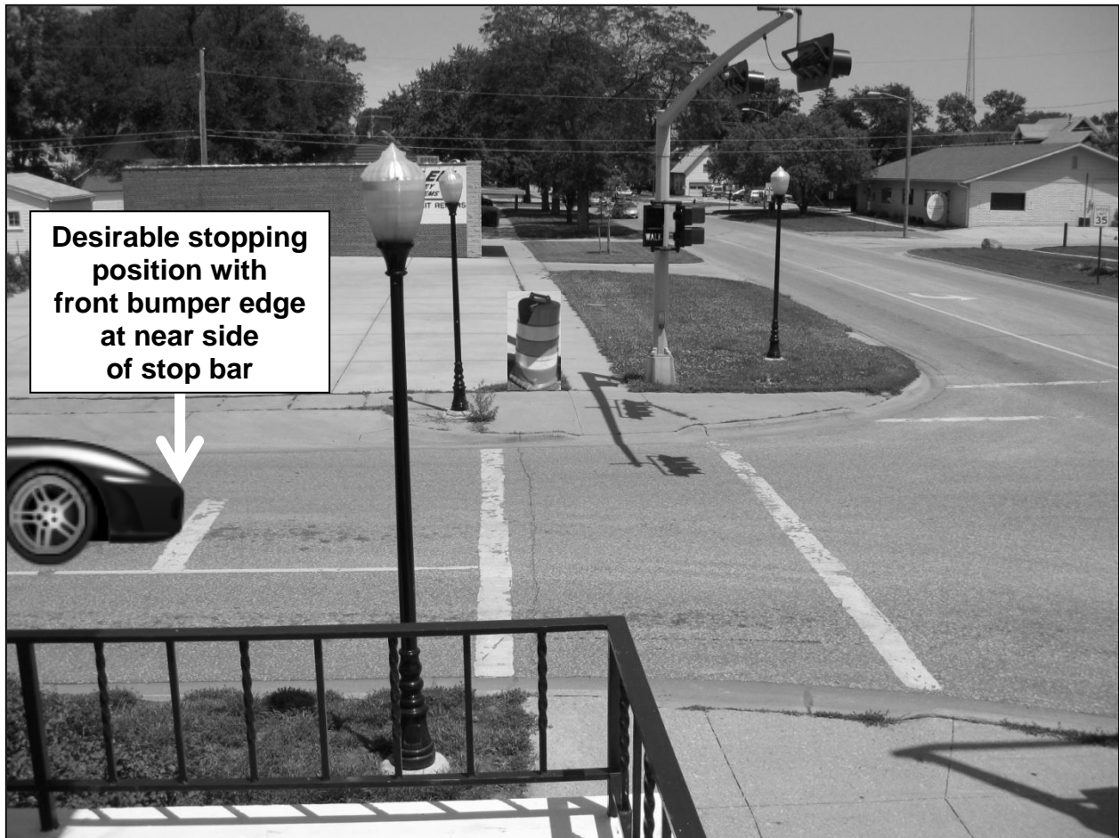
Figure 9.3 View of Staggered Stop Bar on Eastbound Approach to 10 th and Charleston Sts, Lincoln, NE
