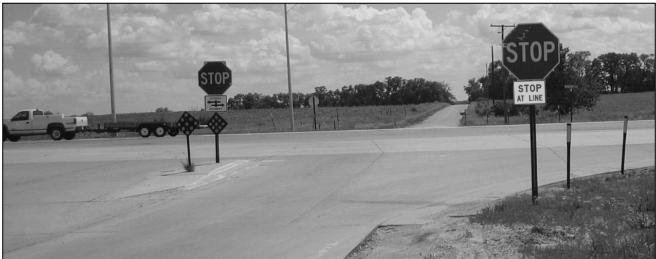
Figure 9.18 Example of Placement of STOP AT LINE Sign Only on Right STOP Sign on ORTL Project
