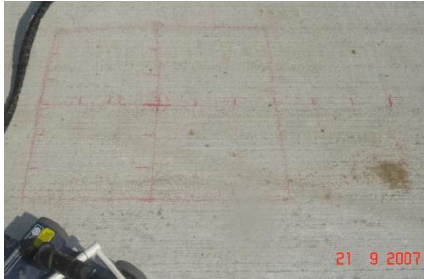
Figure 4.6 Grid used for scan # 1
