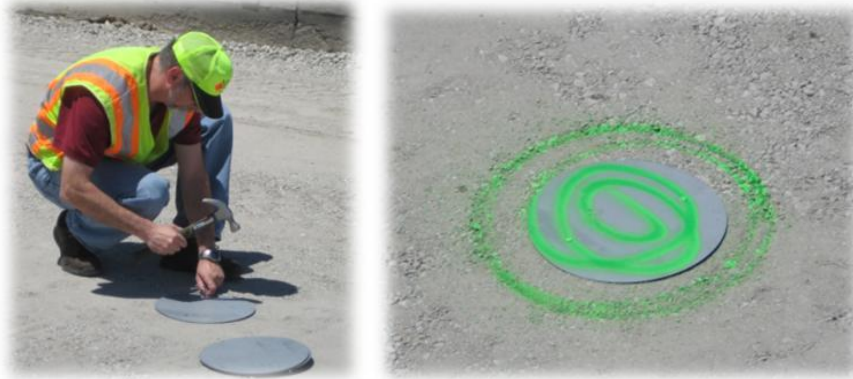
Figure 4.19 Placing reflector disks before paving Hwy 2.
