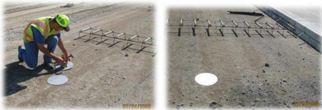
Figure 4.23 Placing reflector disk before paving I-80
