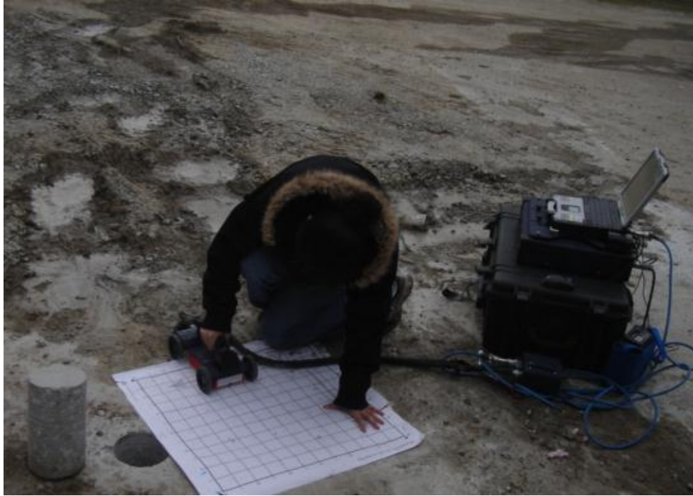
Figure 3.15 GPR grid scan of the test driveway
