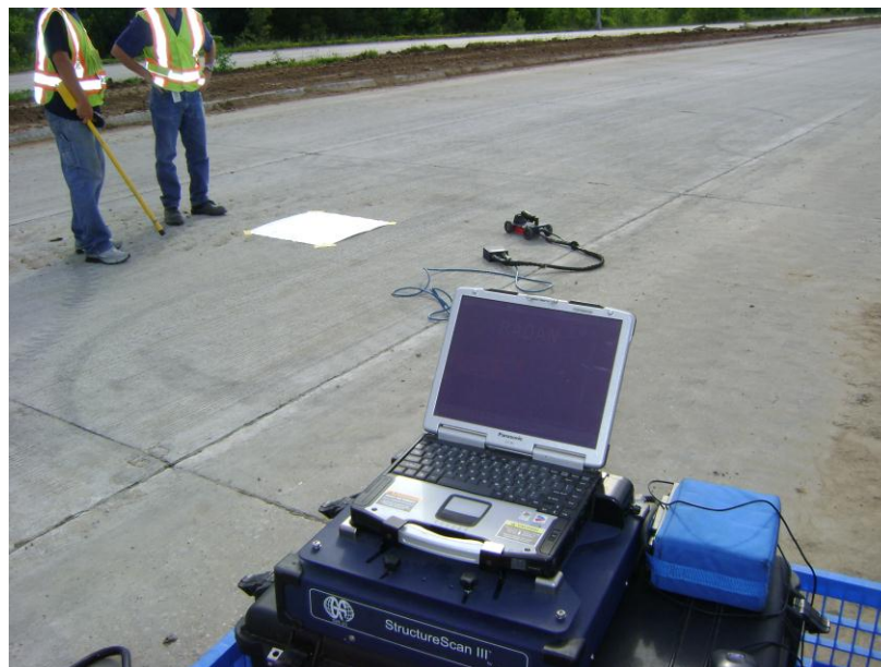
Figure 4.20 Grid scan at the marked location of the steel disk
