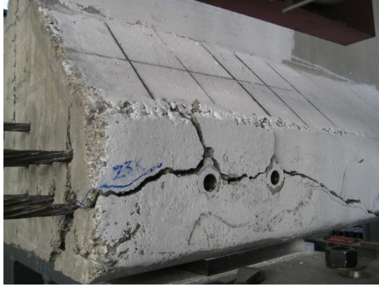
Figure 19: Cracking pattern specimen CB-1.
