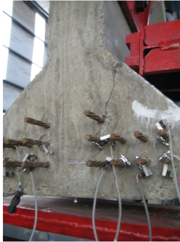
Figure 31: Cracking of specimen HS-3 due to bearing of flange on horizontal actuator loading plate.
