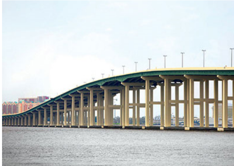
Figure 2: Replacement bridge at Biloxi Bay, MS (B. Hull, MDOT).
