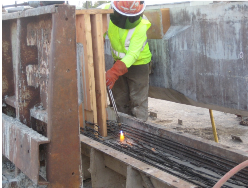
Figure G- 7: Torch Cutting of Prestressing Strand
