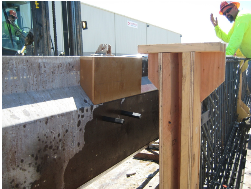
Figure G- 3: Top Flange Blockouts
