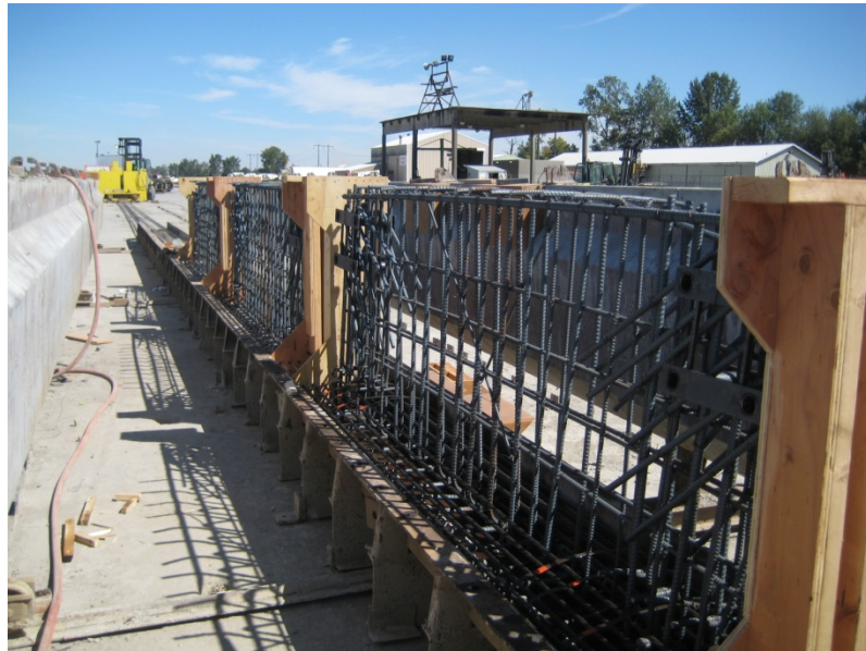
Figure G- 1: Knife River Prestressing Bed
