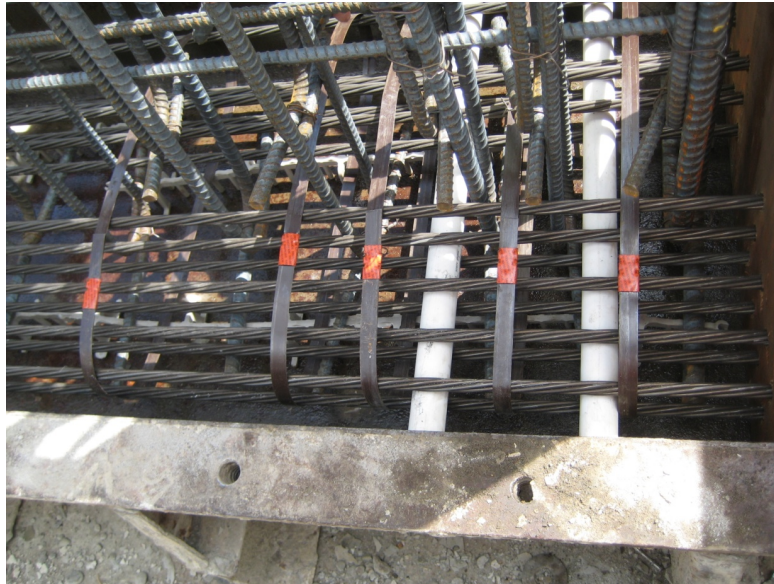
Figure G- 6: Through Bolt (TB) Anchorage
