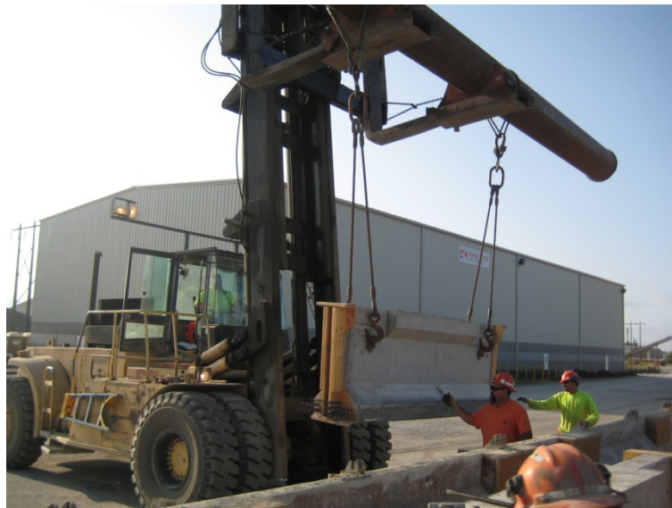
Figure G- 8: Removal of Specimen from Formwork
