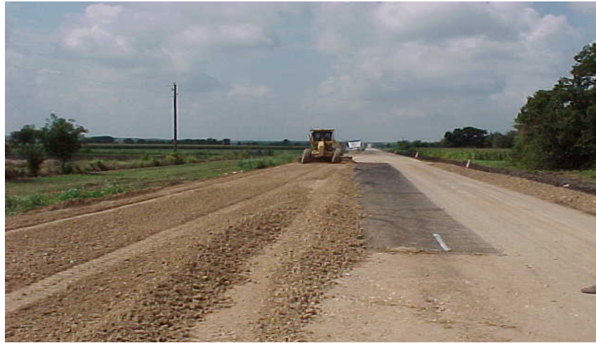
Figure 4.2. Localized Geo-Grid in Potential Problem Location.
