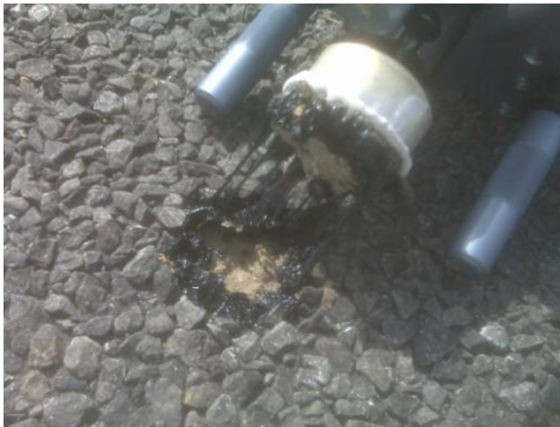
Figure 3.19. Surface Treatment Bond Testing on FM 2502.
