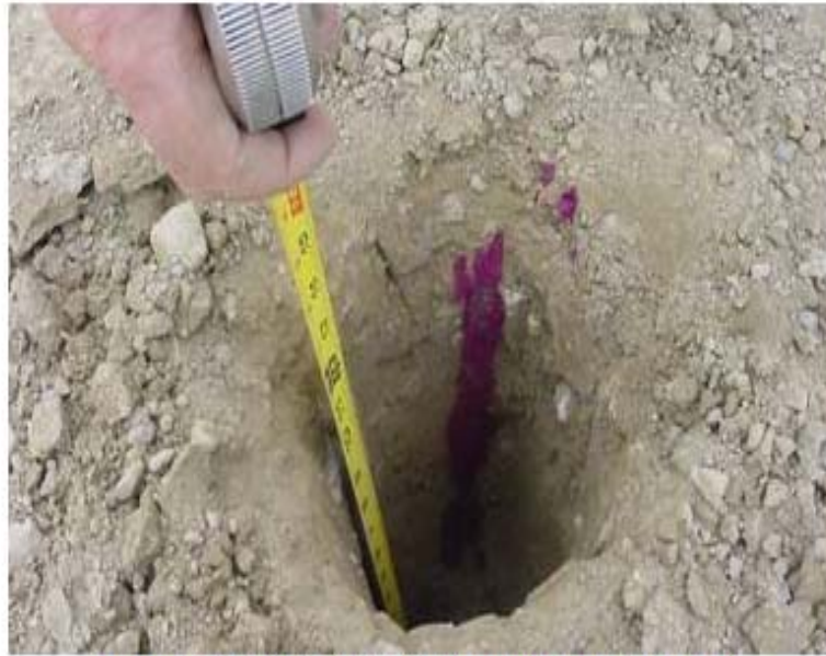
Checking depth of soil stabilization with phenolphthalein
