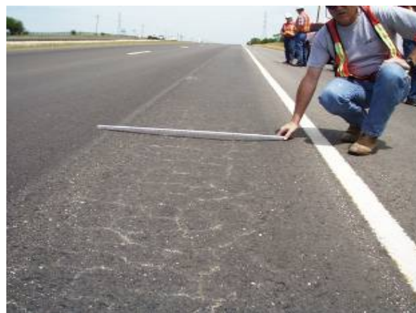
Figure 4.3. Under-Stabilization.
