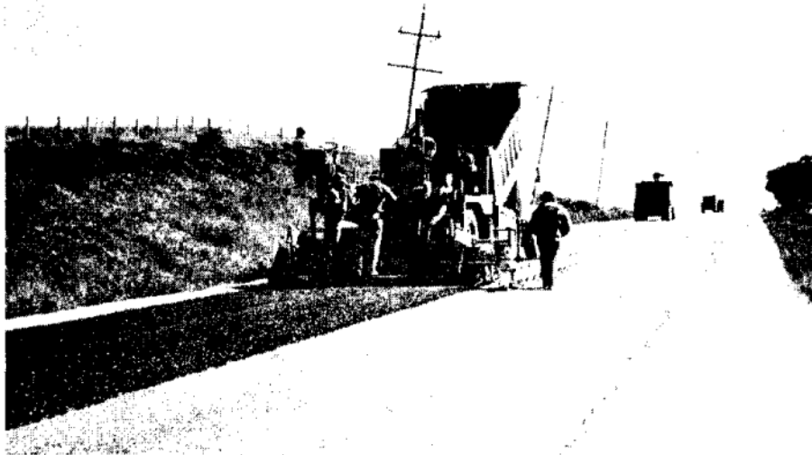
Figure 5 Placement of emulsion treated choke stone
