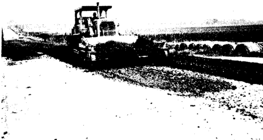
Figure 4 Jersey spreader placing emulsion treated macadam stone
