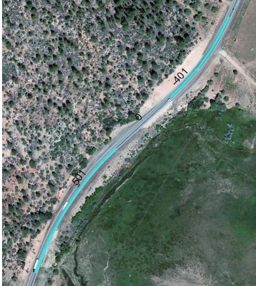
Figure 4-3. Example of short tangent between two curves (radius in feet is shown in black).
