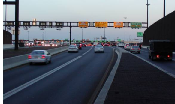
This photo highlights the horizontal and vertical curvature on the approach to the northbound Fort McHenry toll plaza.
