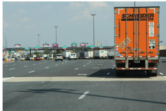
Emergence from the tunnel, horizontal curvature, an uphill grade, and vehicle queues can make wayfinding between the tunnel and toll plaza challenging for drivers.
