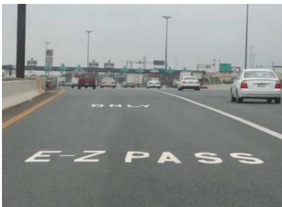
Example of the " E-ZPass ® ONLY" pavement markings and solid white stripe (toll lane 11, approach lane D).
