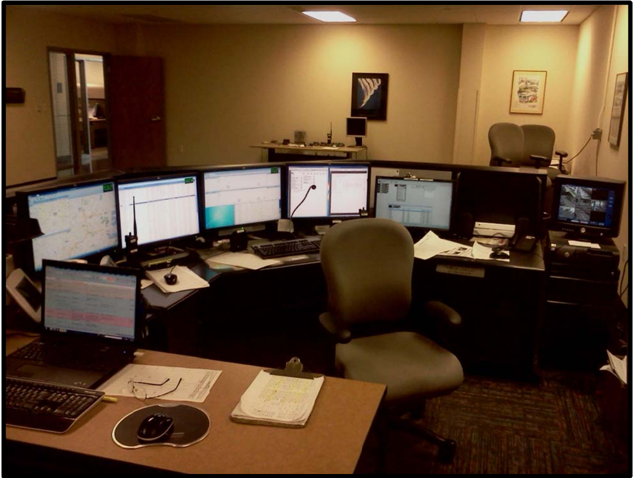
Figure 3-2 Radio Control Room – South County Station
