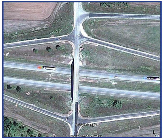
I-70 K-14 West interchange (Google photo).
