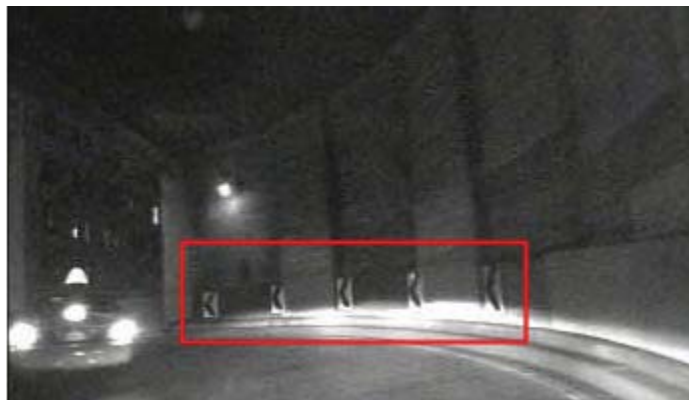
Figure 68: Left Curve Inside a Tunnel
