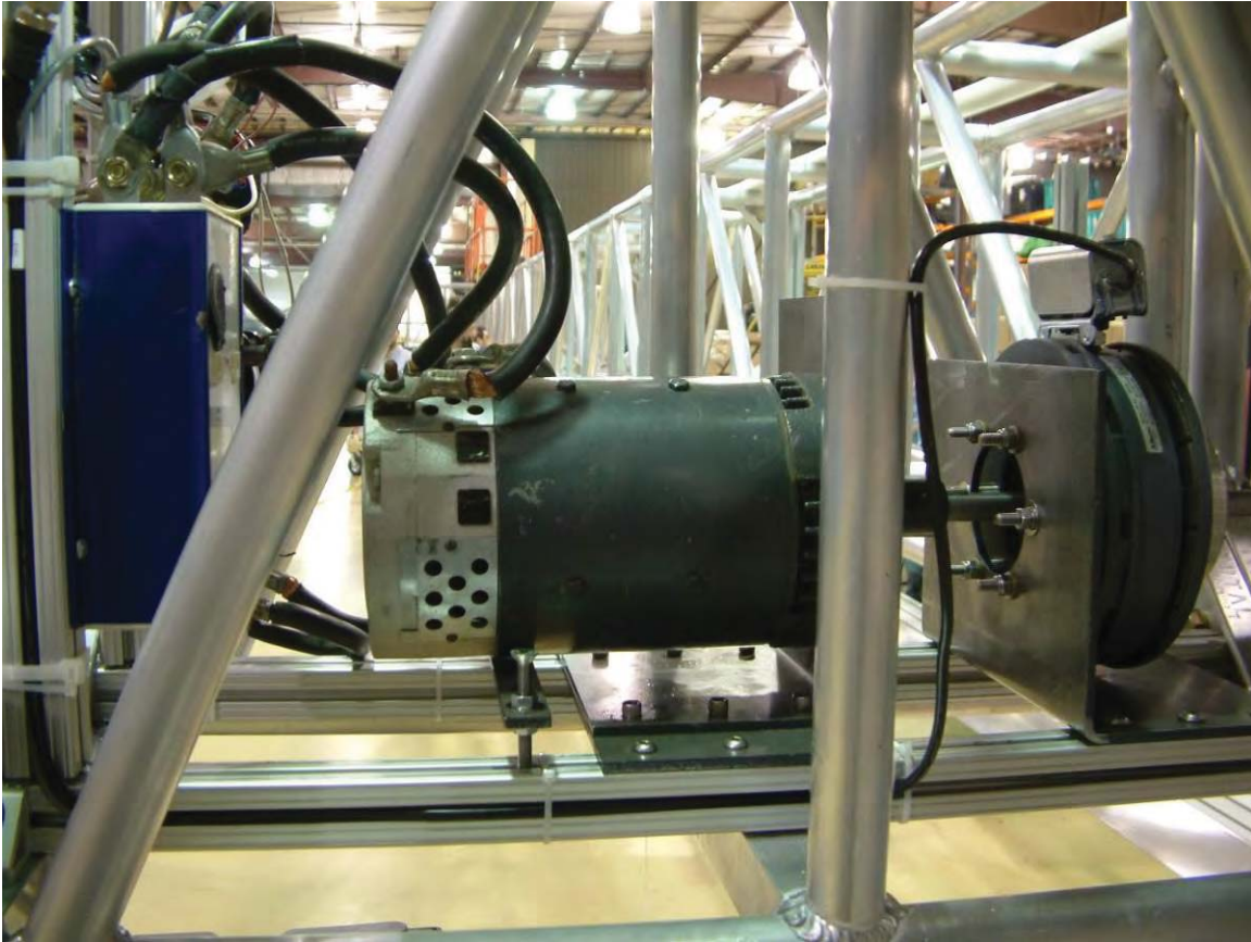
Figure 180: Illustration of Motor Controller (left), Motor (center) and Brake (right)
