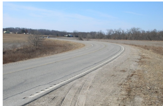
Figure B-2. Rumble stripe installation on F-29 (courtesy of Bob Sperry, InTrans)
