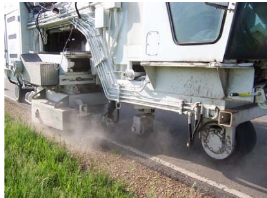
Figure B-1. Close-up of the milling process (courtesy of Bob Sperry, InTrans)
