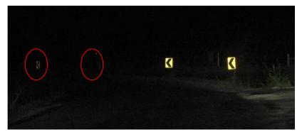
When signs are out of proper alignment, they will not be as visible at night.
