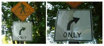
Signs under a tree canopy are often covered with mold (left photo) which can easily be cleaned (right photo, right half of sign).
