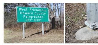
I-beam steel posts with a slip base are needed for larger roadside guide signs.
