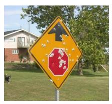
Signs with extensive gunshot holes should be replaced.
