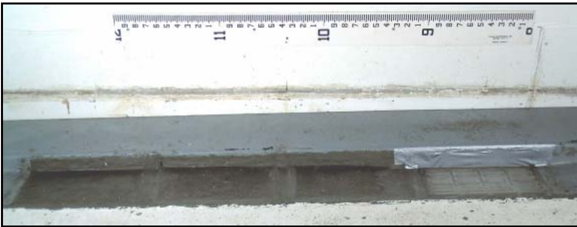
Figure 3.11 Single No. 13 Combination with Grate Only Photograph
