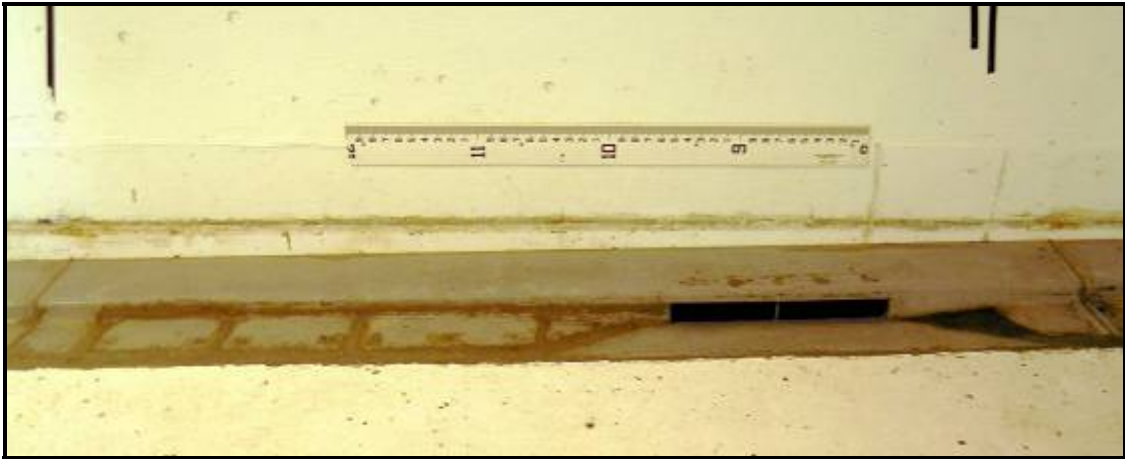
Figure 3.22 R5 Curb Inlet Photograph
