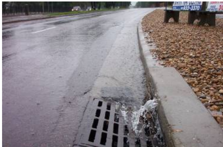
Figure 7.1 Splash-Over Flow Over Type 13 Grate
