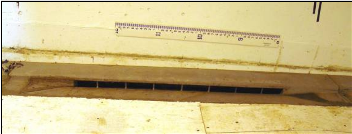
Figure 3.25 R15 Curb Inlet Photograph
