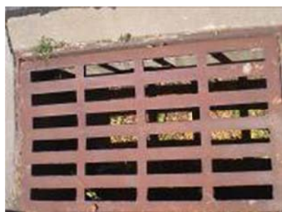
(a) grate inlet
