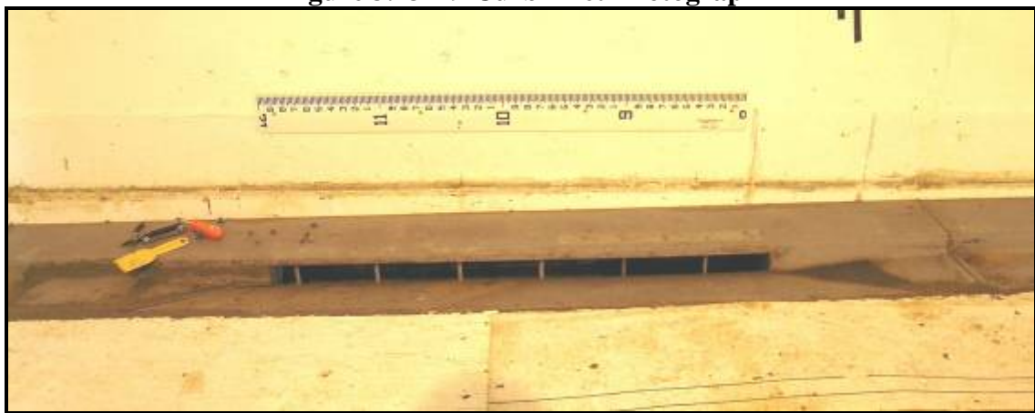
Figure 3.24 R12 Curb Inlet Photograph
