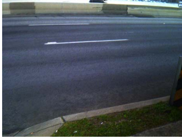
Figure 65. Replaced Site IH10Fr.
