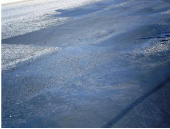
Figure 55. Various 2/10 Patches on Site IH10Fr.
