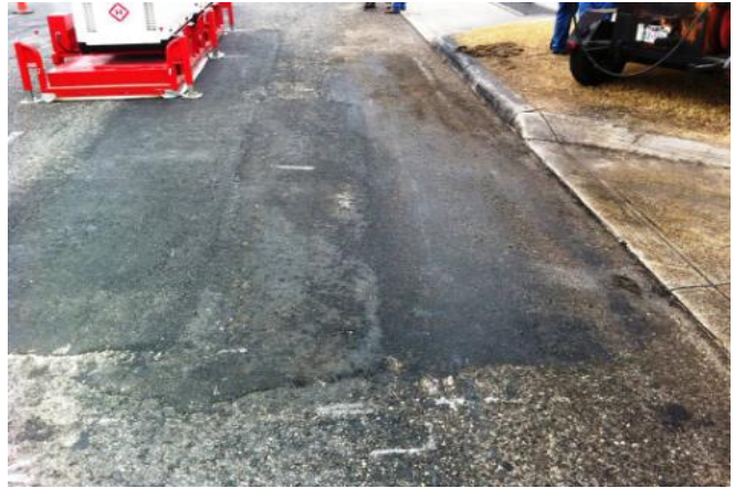
Figure 23. Multiple Patches and Overlap.
