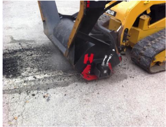
Figure 14. Milling and Scarifying.
