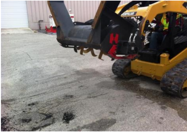
Figure 13. Preparing to Mill and Scarify.
