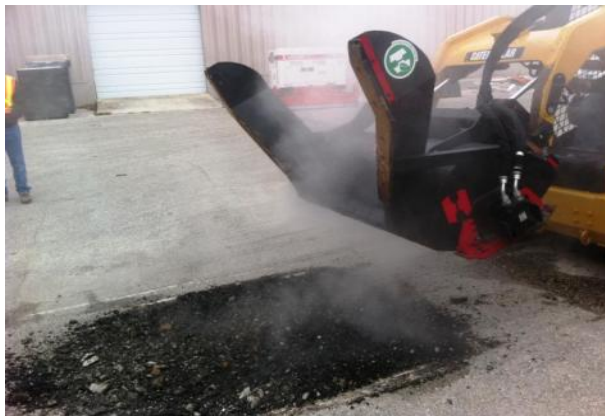
Figure 16. Preparing to Mill and Scarify.
