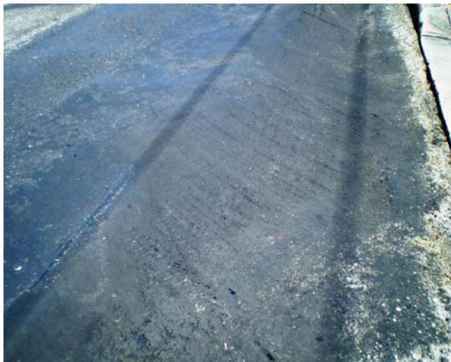
Figure 51. Patches 2/10-4 and 7 on Site IH10Fr.
