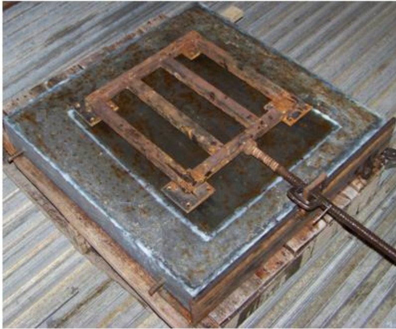
Figure 3.10 Applying acrylic sealant on concrete slab
