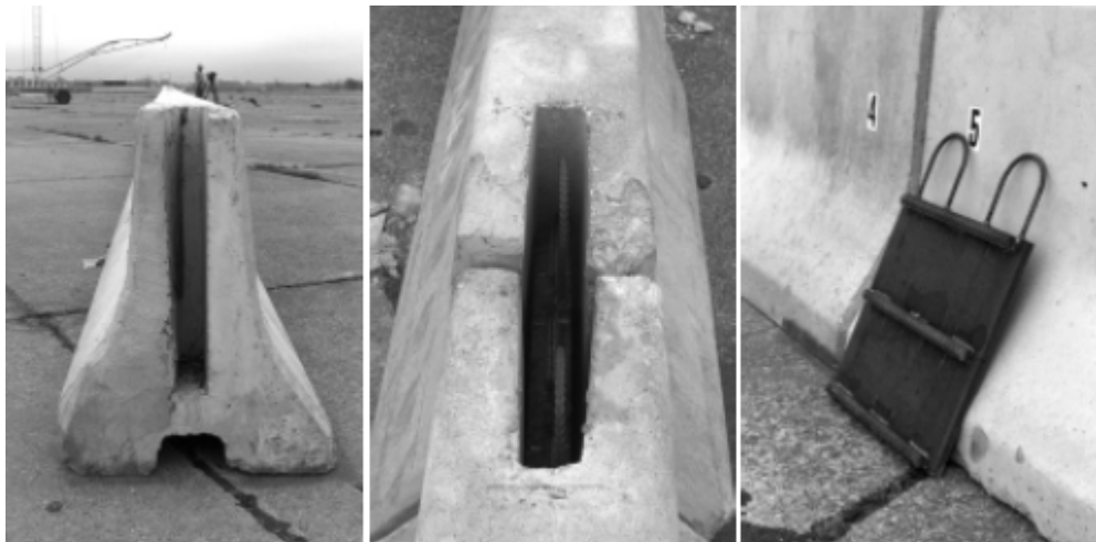
Figure 8: Texas grid-slot connection (Bligh et al., 2002)
