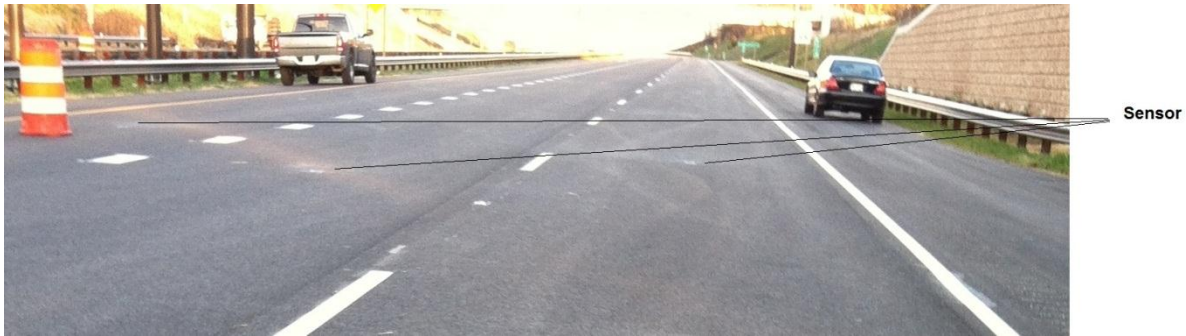
Figure 23. Test segment of the Inter County Connector after sensor installation
