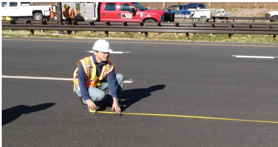
Figure 21. Measuring and marking the location of sensors for installation
