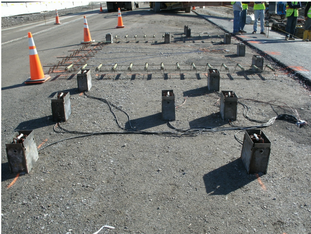
Figure 10 Sensors are enclosed in metal boxes during paving to prevent damage
