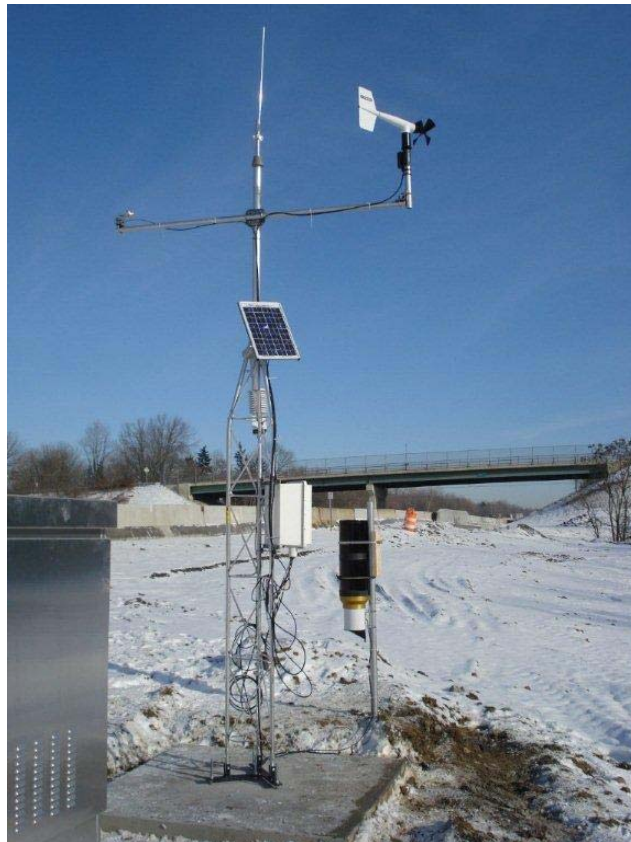
Figure 9 Weather station at mile marker 300 along I-90
