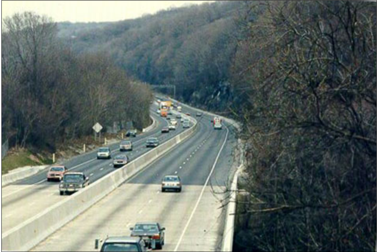
Figure 1. Concrete Median Barrier on a Narrow Median Suburban Highway with High Traffic Volume
