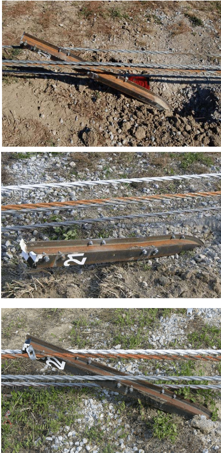
Figure 43. Post Nos. 20-22 Damage, Test No. 4CMB-1
