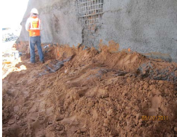
Figure 9.19. Shotcreting the Exterior Soil Face.
