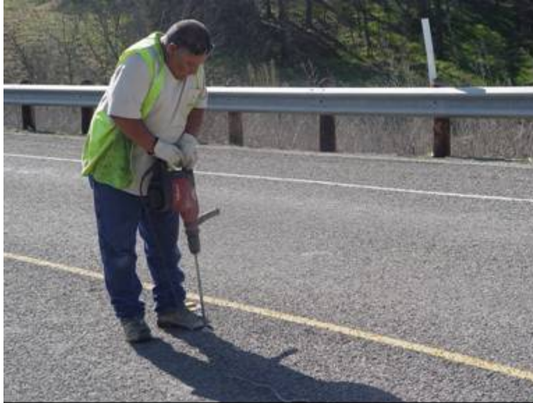
Figure 9.6. Drilling Holes into the Approach Slab.
