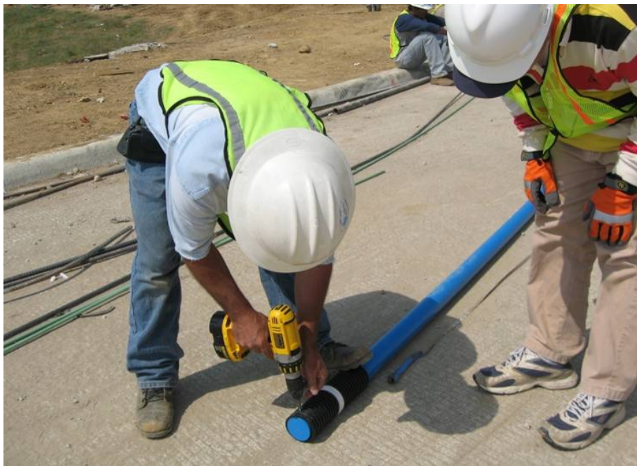
Figure 6.15. The Bottom of the Casing Was Plugged with a Bottom Cap.
