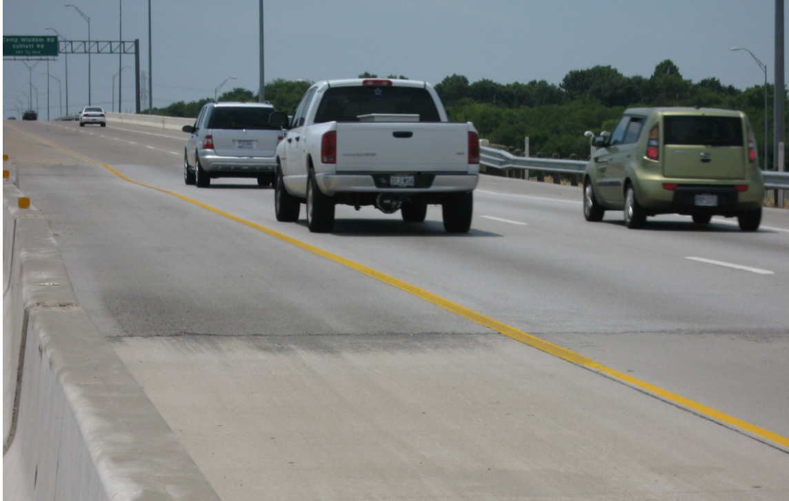
Figure 7.28. Bridge Approach in the Control Section Overlaid by Hot Mix Asphaltic Concrete to Mitigate the Bump.
