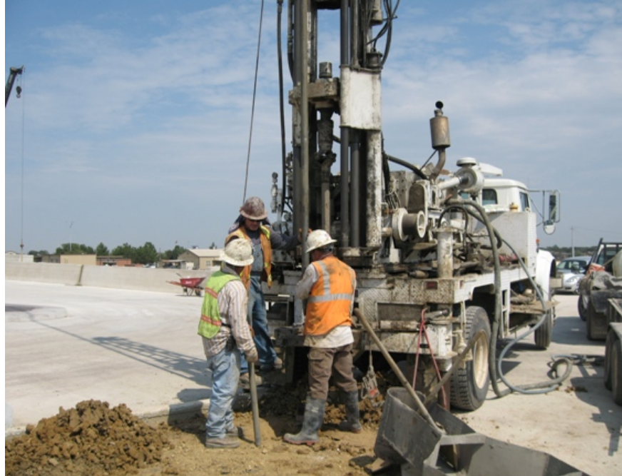
Figure 6.14. A Selected Location Was Bored to Install the Inclinometer Casing.
