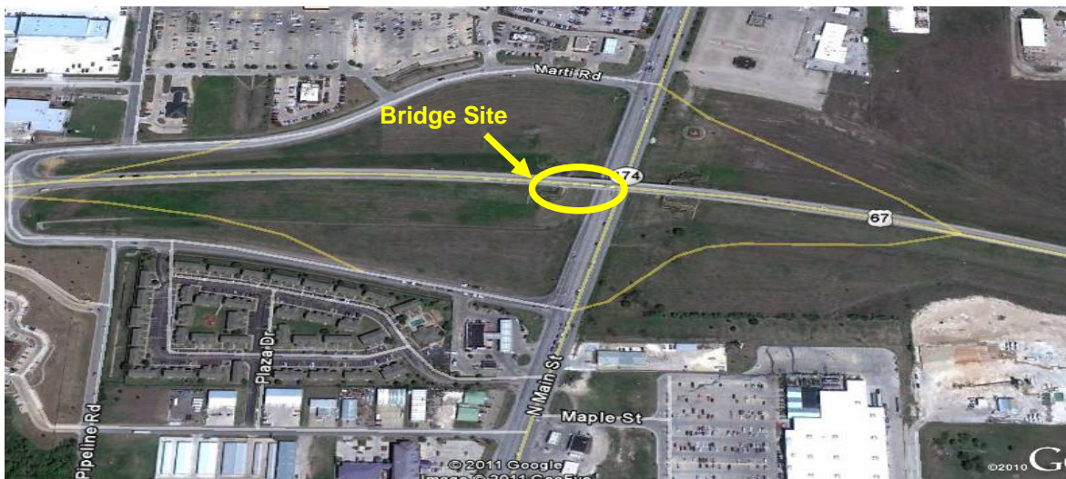
Figure 9.13. Bridge Site at US 67 over SH 174.
