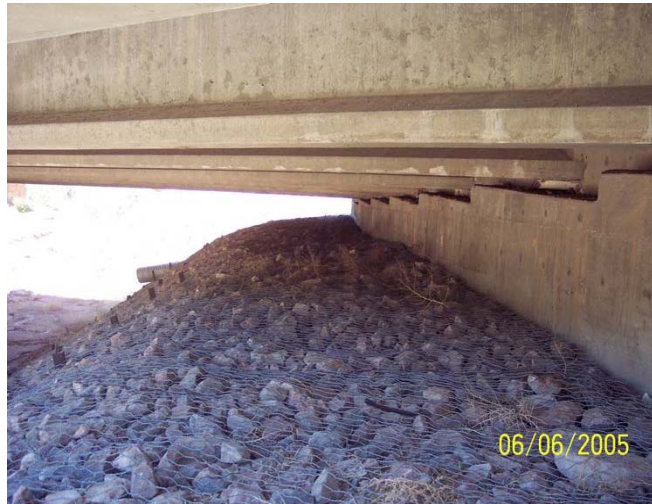
Figure 2.58. Riprap Used for Erosion Control (Lenke, 2006).
