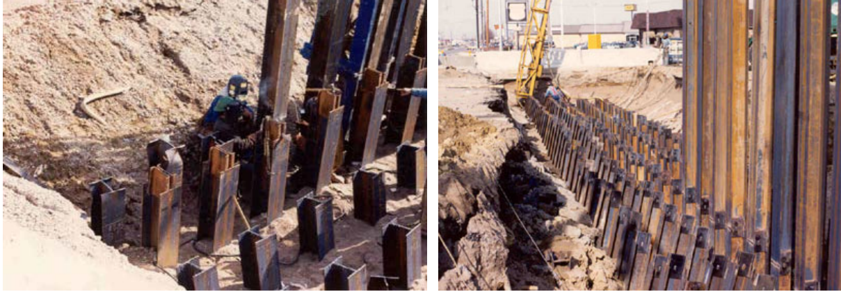
Figure 2.43. Example of Bridge Foundation Using Steel H-Piles.
