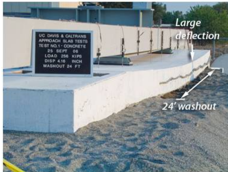
Figure 2.63. Simulated Approach Slab Deflection due to Washout by UC Davis Research Team.
