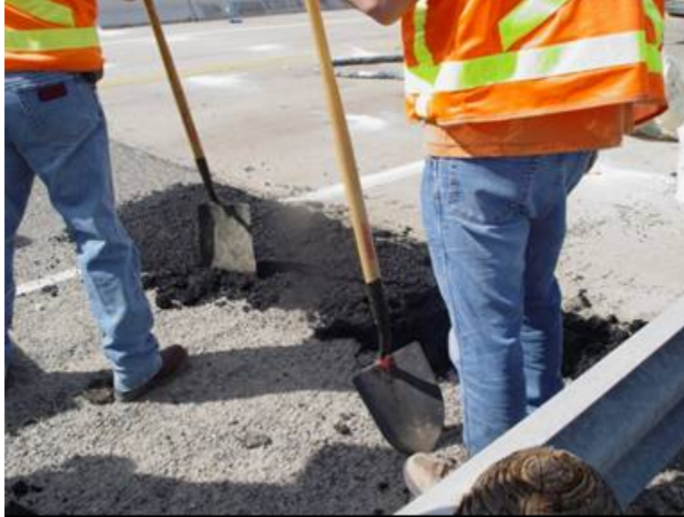
Figure 9.12. Level-Up of Uneven Sections with Cold Asphalt Mix.
