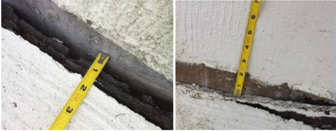
Figure 7.27. Opening Observed close to the Abutment of the Bridge.
