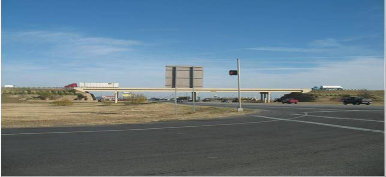
Figure 9.14. Existing Bridge along US 67 Crossing over SH 174.
