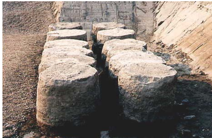
Figure 2.28. Deep Soil Mixing (DSM) Operation and Extruded DSM Columns.
