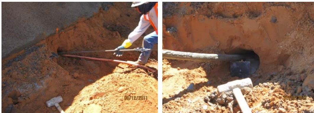
Figure 9.18. Placing of Nails and Grouting the Holes.
