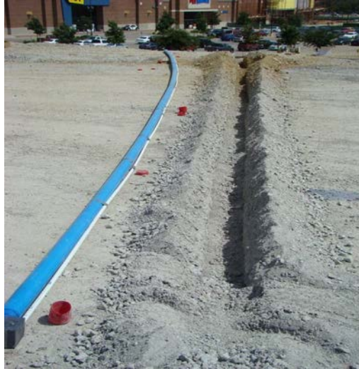
Figure 6.21. A Trench Was Excavated at the Selected Location.
