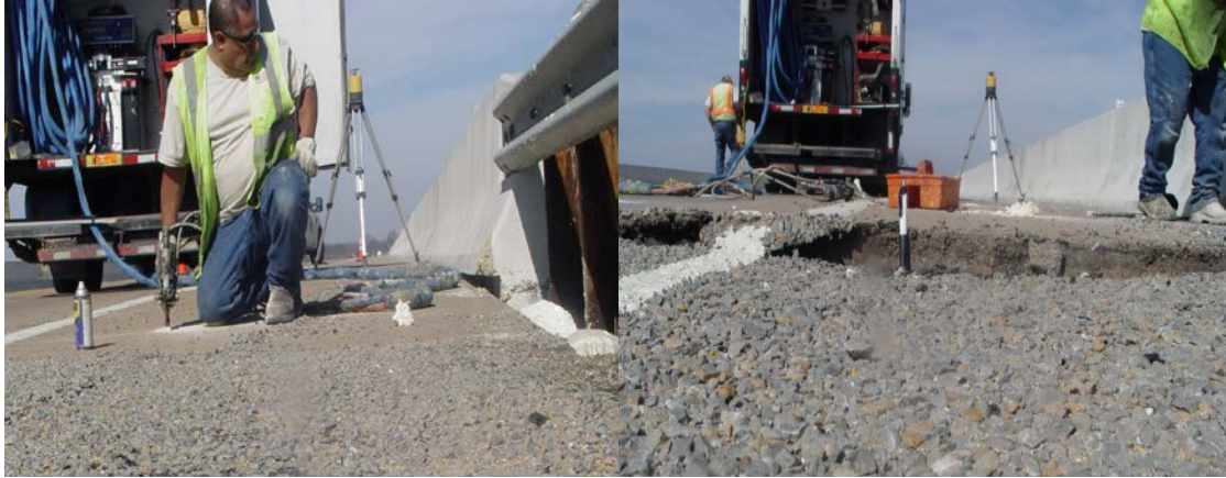
Figure 2.67. Position of Approach Slab during and after the Urethane Foam Injection Process.
