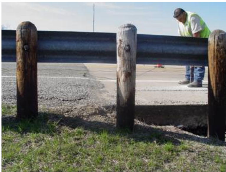
Figure 9.7. Another View of Drilling Holes.
