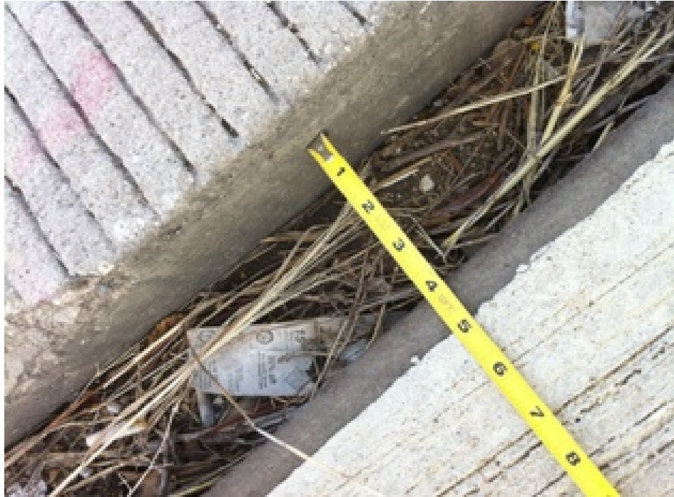
Figure 7.24. Lateral Movement of the Platform around Inclinometer V4.
