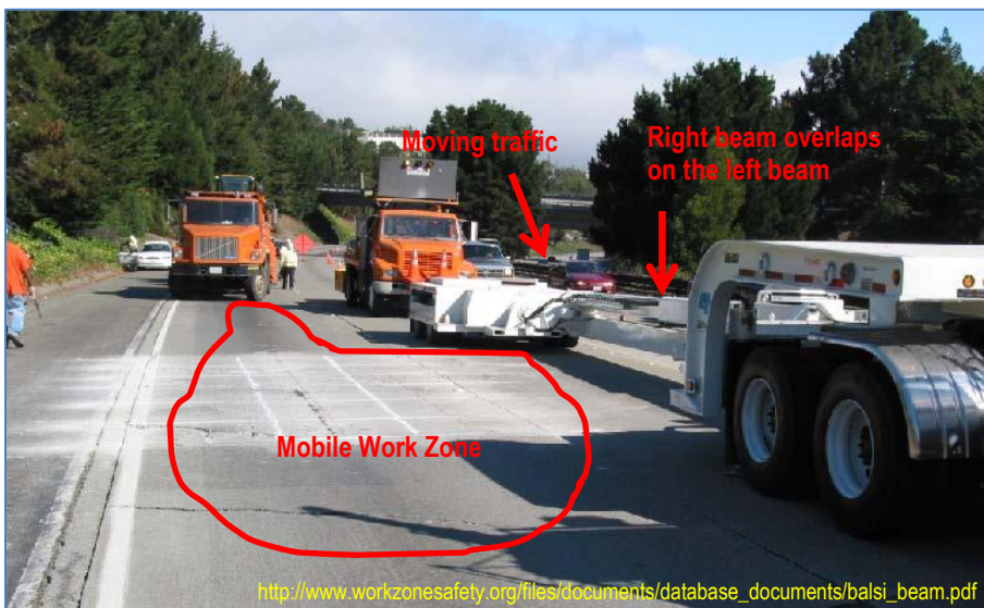
Figure D.3. Final stage: the two beams are overlapped on one side
