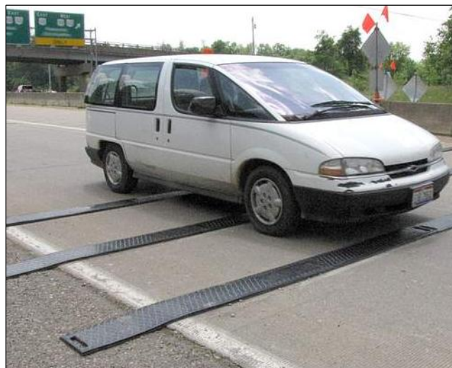
Figure C.6. Temporary rumble strips
