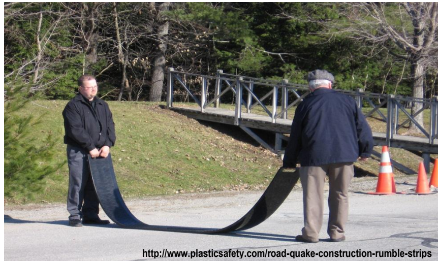
Figure D.11. Two people placing portable rumble strips
