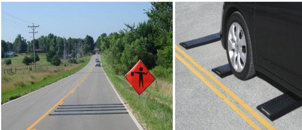
Figure 3. Flagger stopping traffic (left) and portable temporary rumble strips being field tested near Perry, Kansas (right)
