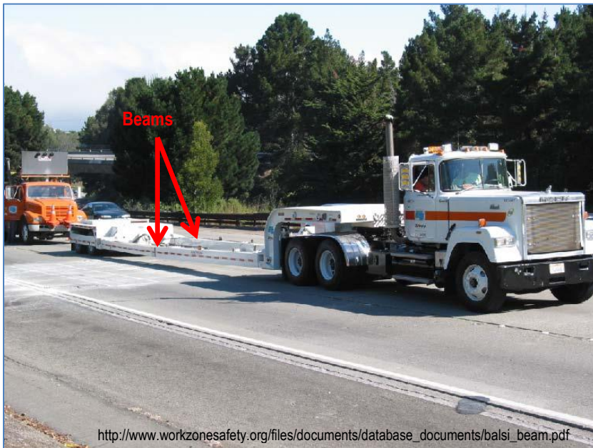
Figure D.1. First stage of Balsi Beam installation at worksite
