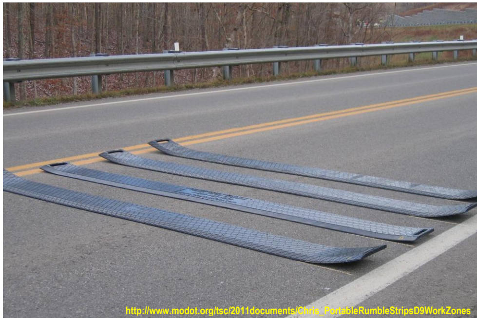
Figure D.10. Portable rumble strips
