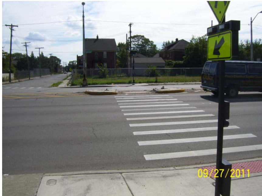
Photo of Davison Avenue at Lawton Avenue pedestrian refuge island
