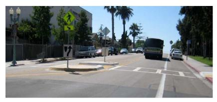
thermoplastic pavement markings and continental "ladder style" crosswalk markings. Highly visible continental style crosswalk markings are recommended at midblock and uncontrolled intersection locations.
