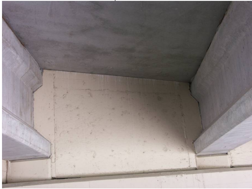
Figure 6-2. Backwall-abutment connection details
