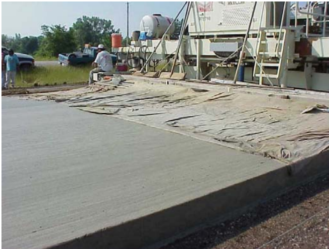
Figure 2.3. Burlap drag method
