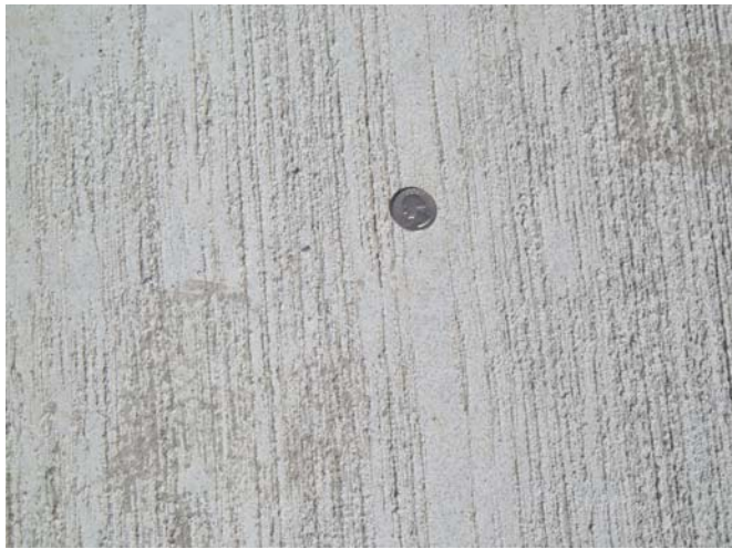
Figure 2.2. Artificial turf drag texture
