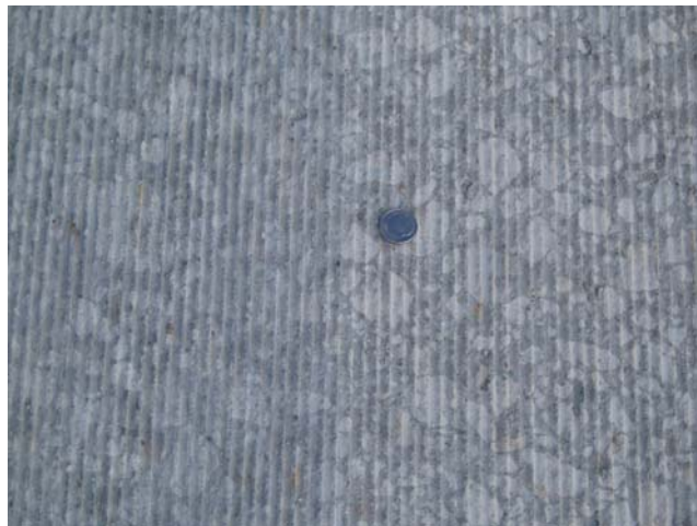
Figure 2.9. Texture after diamond grinding
