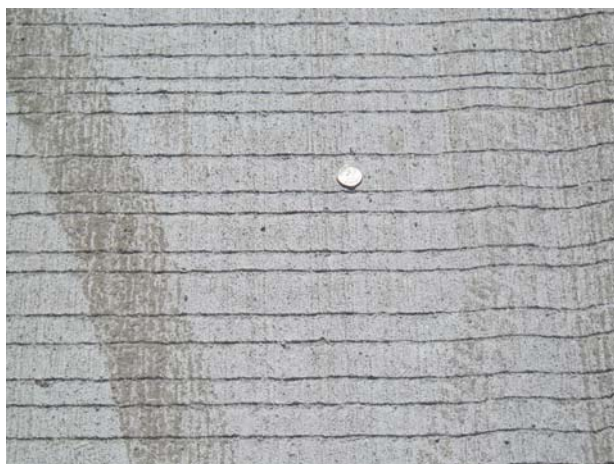
Figure 2.6. Transverse tining—randomly spaced
