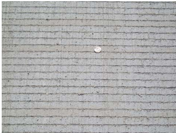
Figure 2.5. Transverse tining—uniformly spaced
