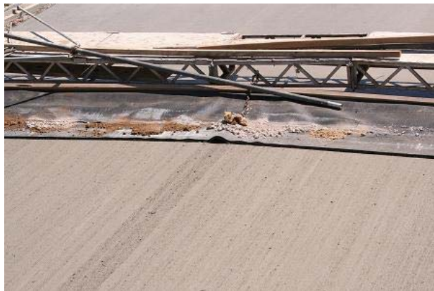
Figure 2.1. Artificial turf drag method
