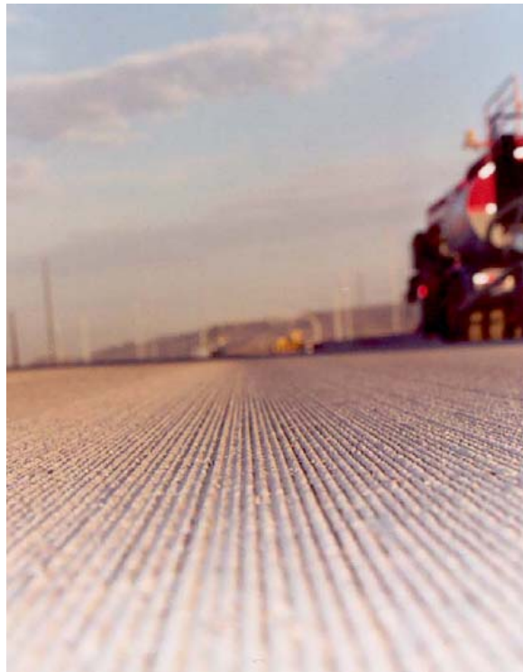
Figure 2.8. Diamond ground pavement
