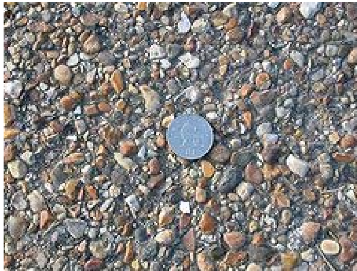
Figure 3.2. Finished exposed aggregate surface
