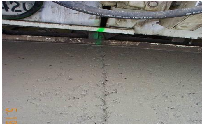
Figure 2.2.9.3 Knife Formed Joint (Steffes, 2005)
