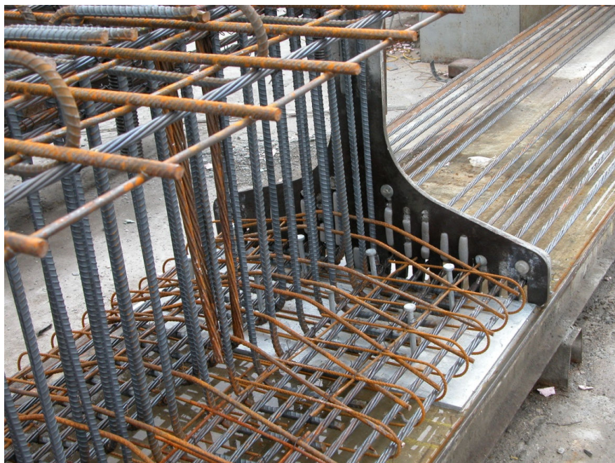
Figure 3.3.3: Common End Plate
