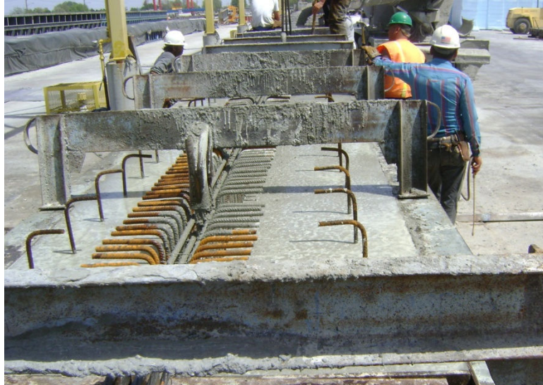
Figure 4.3.8: Pouring of concrete
