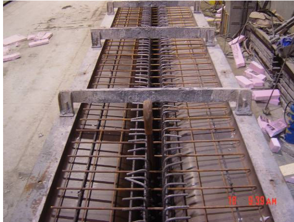
Figure 2.5.4: Top reinforcement
