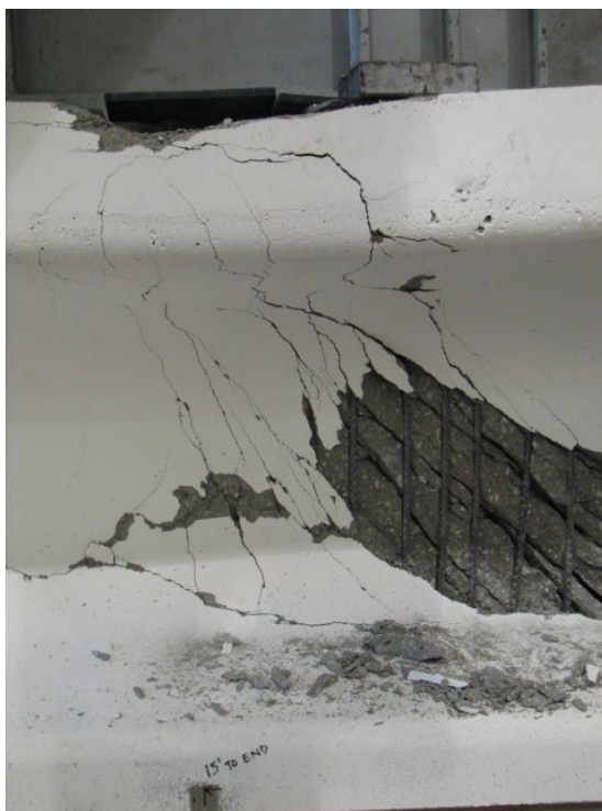
Figure 2.11.4.7: Flexure cracking at load point
