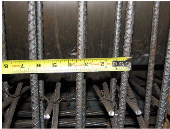
Figure 2.5.2: Typical shear reinforcement, #4 at 3 in spacing
