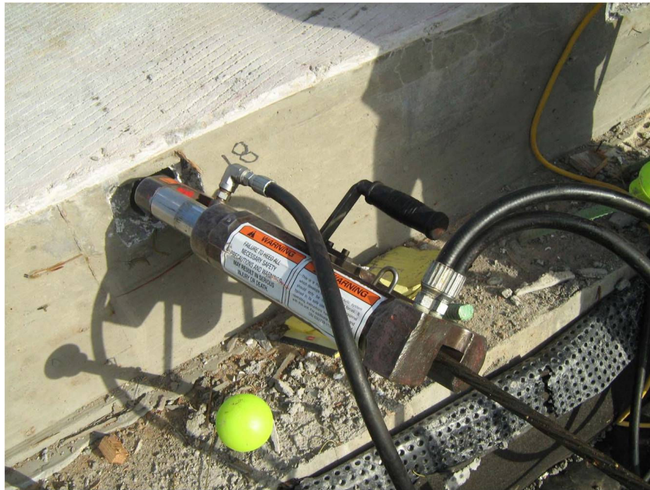
Figure A.6: Post tensioning jack
