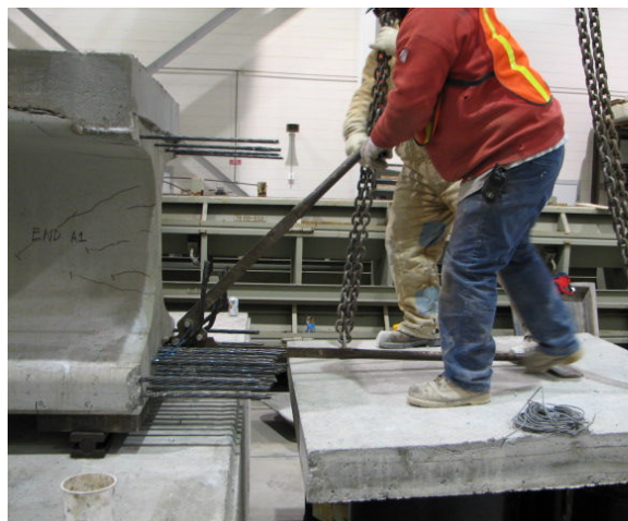
Figure 2.10.1: First 45 degree strand bend
