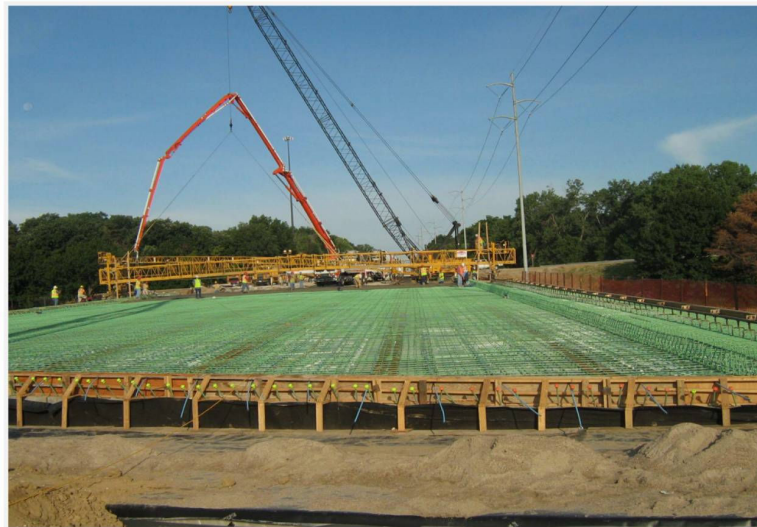
Figure A.5: Bridge construction
