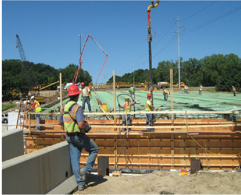
Figure A.12: Pouring of Concrete
