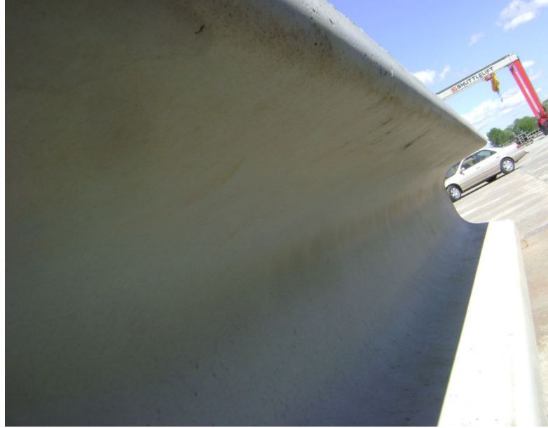
Figure 4.3.10: Girder after release
