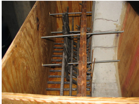
Figure 2.10.4: Diaphragm reinforcement
