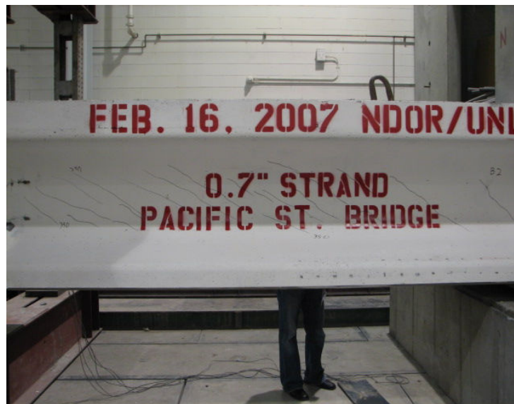
Figure 2.11.4.3: Shear cracking in the web
