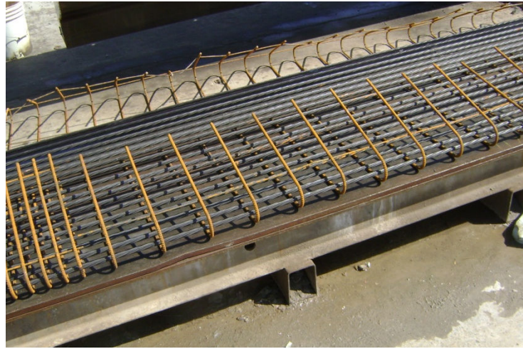
Figure 4.3.6: Placement of confinement reinforcement
