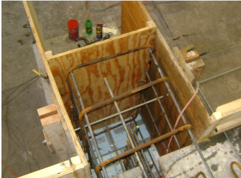
Figure 4.4.11: Formwork around diaphragm
