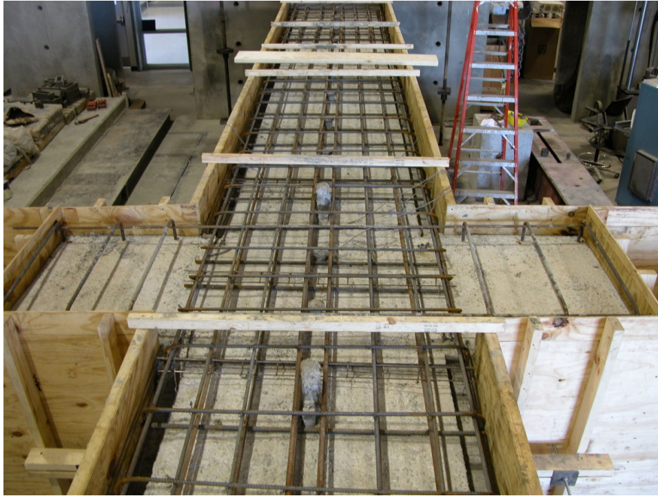
Figure 3.3.15: Place Deck Reinforcement
