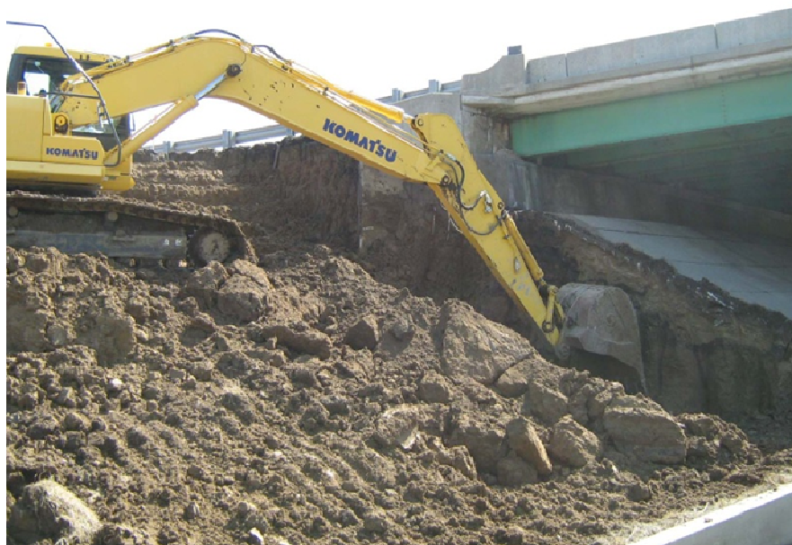
Figure A.7: Excavation
