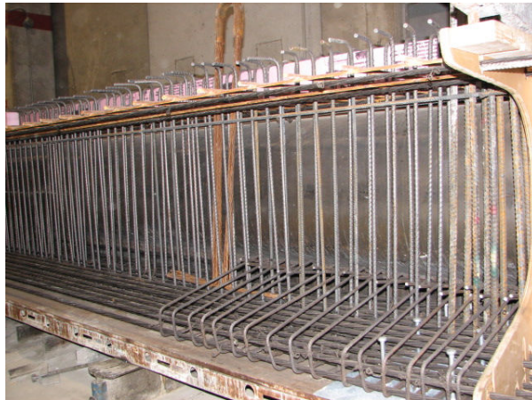
Figure 2.5.1: Shear and confinement reinforcement
