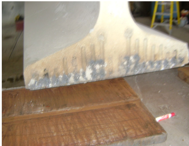
Figure 4.4.2: 2 inch bearing plates
