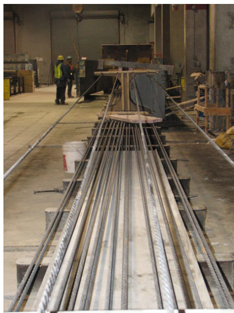
Figure 2.4.2.3: Strand profile adjustment to specified pattern
