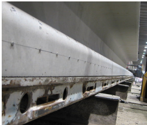
Figure 2.9.2: DEMEC point placement and camber
