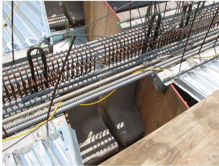
Figure A.4: Girders at diaphragm section
