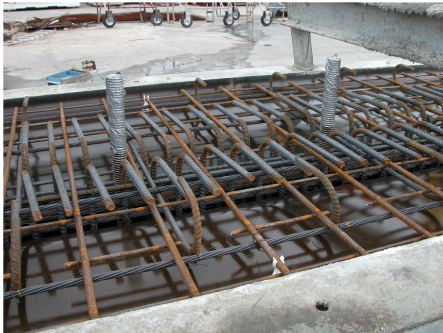
Figure 3.3.1: Confinement at the End of the Girder and C shape Bar around TR
