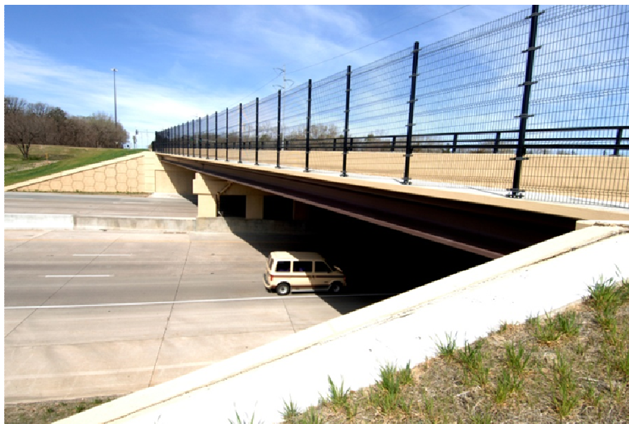
Figure A.14: Completed bridge
