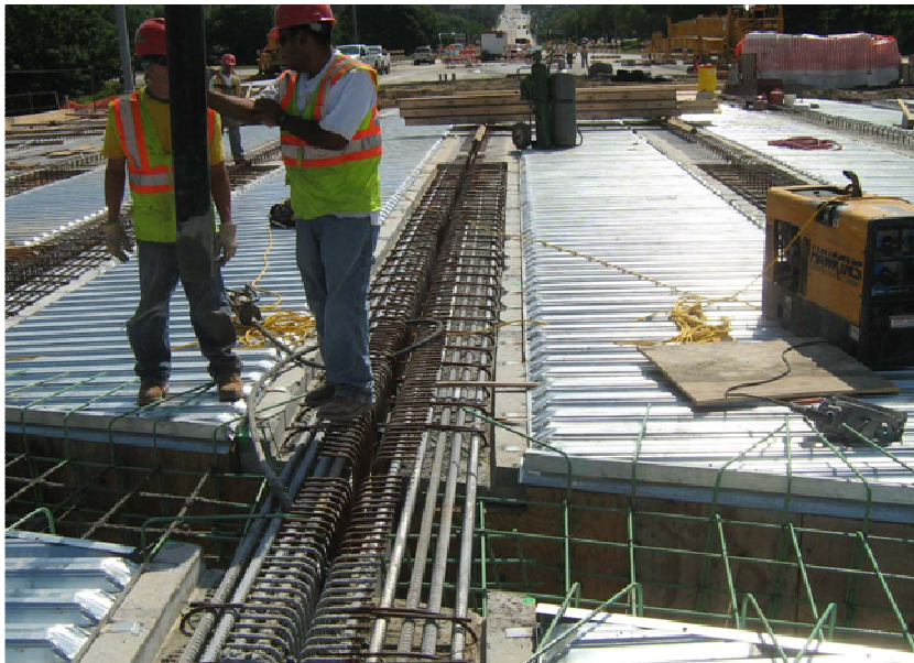
Figure A.11: Pouring of Concrete
