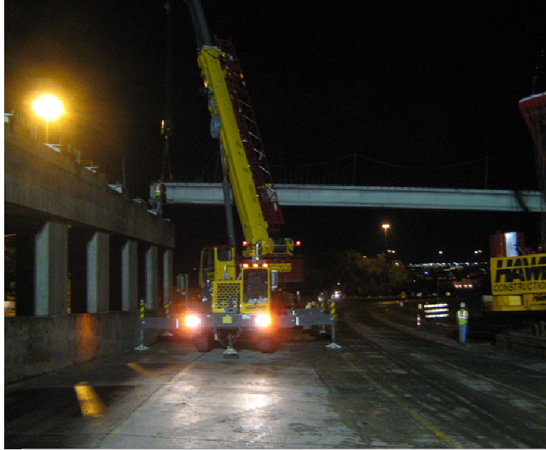
Figure A.10: Bridge Construction
