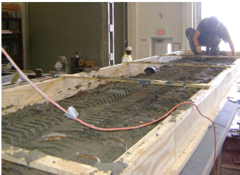
Figure 4.4.14: Pouring of 3.5 inch interface block
