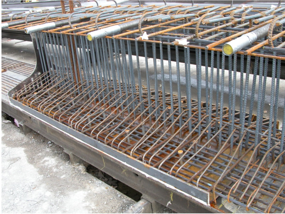
Figure 3.3.1: Confinement at the End of the Girder and C shape Bar around TR
