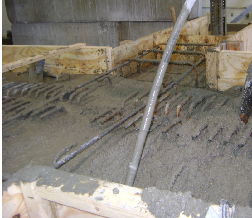
Figure 4.4.13: Pouring of diaphragm
