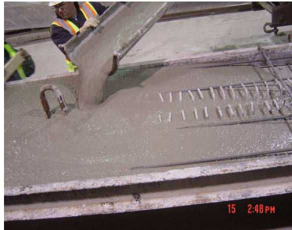
Figure 2.8.2: Pouring the deck
