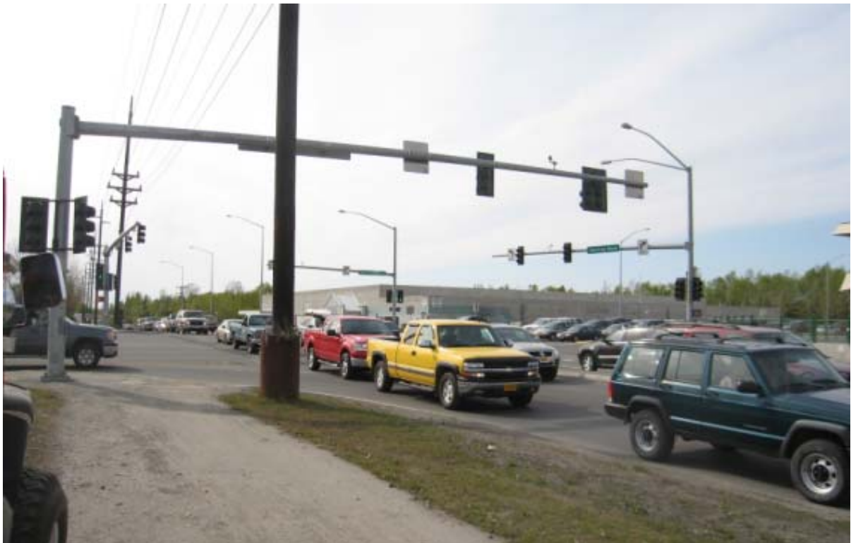
Figure 3 Picture showing the queue from the eastbound entrance approach blocking the upstream intersection at Old Seward Highway/E. Dowling Road
