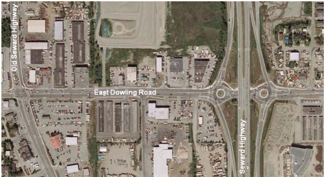
Figure 1 East Dowling Road Roundabouts (Source: Google Maps®)
