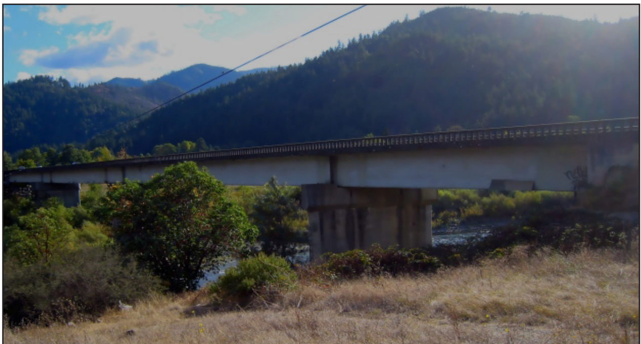
Figure 25. The Trinity River Bridge Underpass
