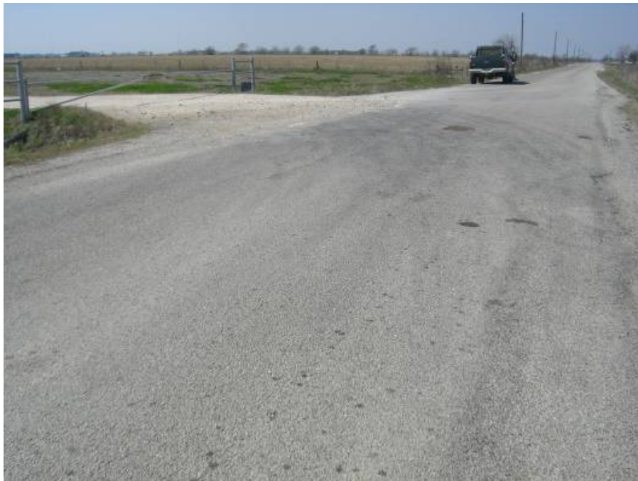
Figure 97. County Road to Saltwater Disposal Facility (2).
