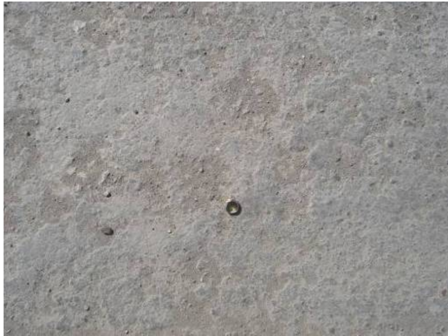
Figure 93. Oakridge Ranch Private Road (Road Surface).
