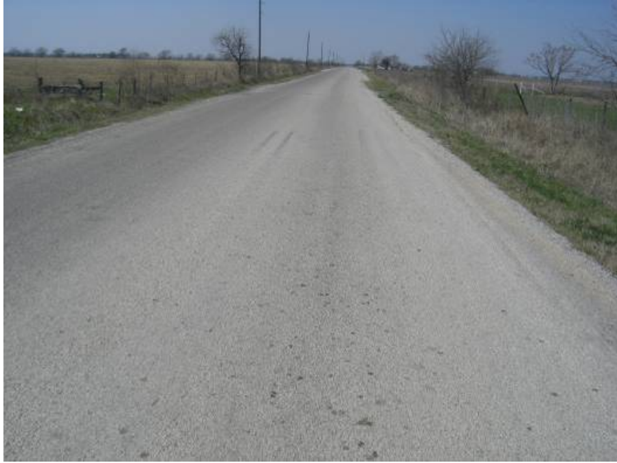
Figure 96. County Road to Saltwater Disposal Facility (1).
