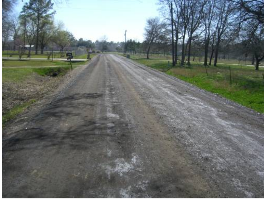
Figure 95. Greenbriar County Road, Primed with MC-30 (2).
