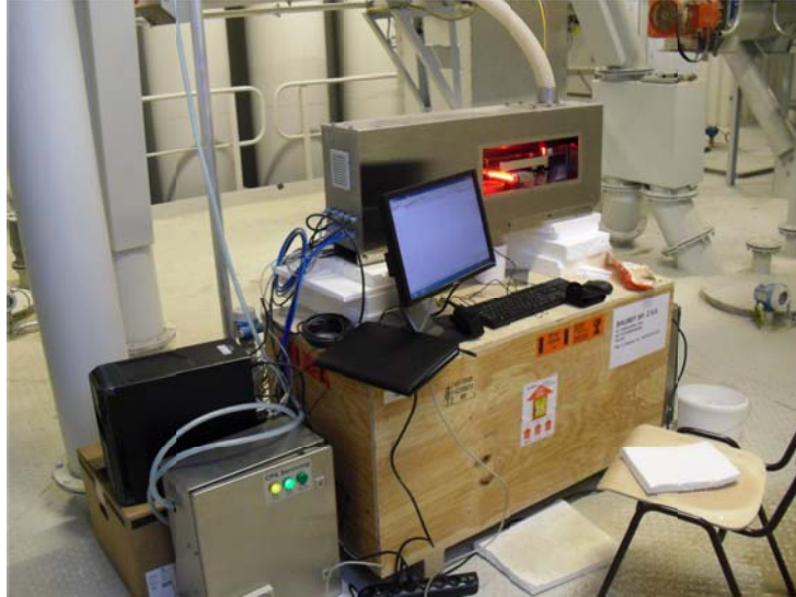
Figure 13 CPA On-Line System at a Building Construction Materials Production Facility in Poland
